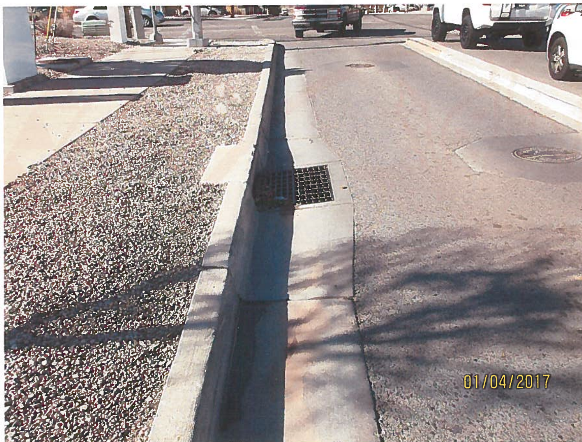
Sediment entering inlet in Holly Ave.
