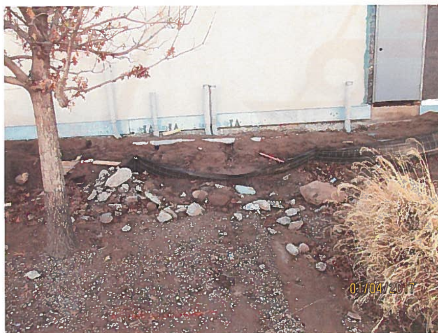
Silt fence down.
