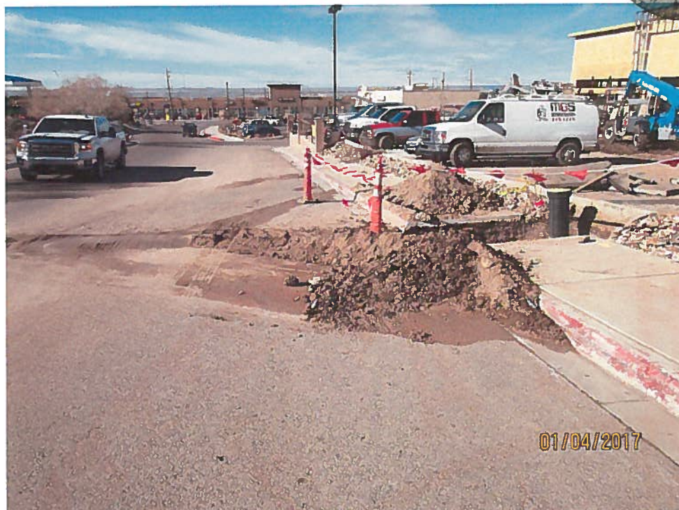
Unprotected dirt pile in access road with recent waterline work.
