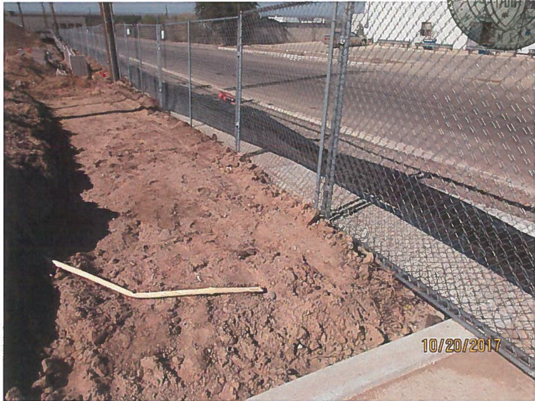
Silt fence not buried.
