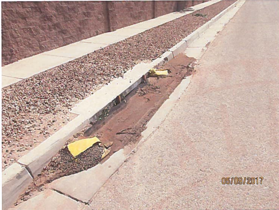
Inlet protection on Oakland requires maintenance.
