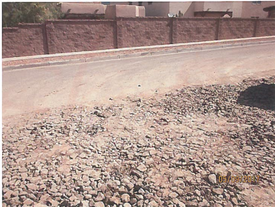
Track-out pad requires maintenance.
