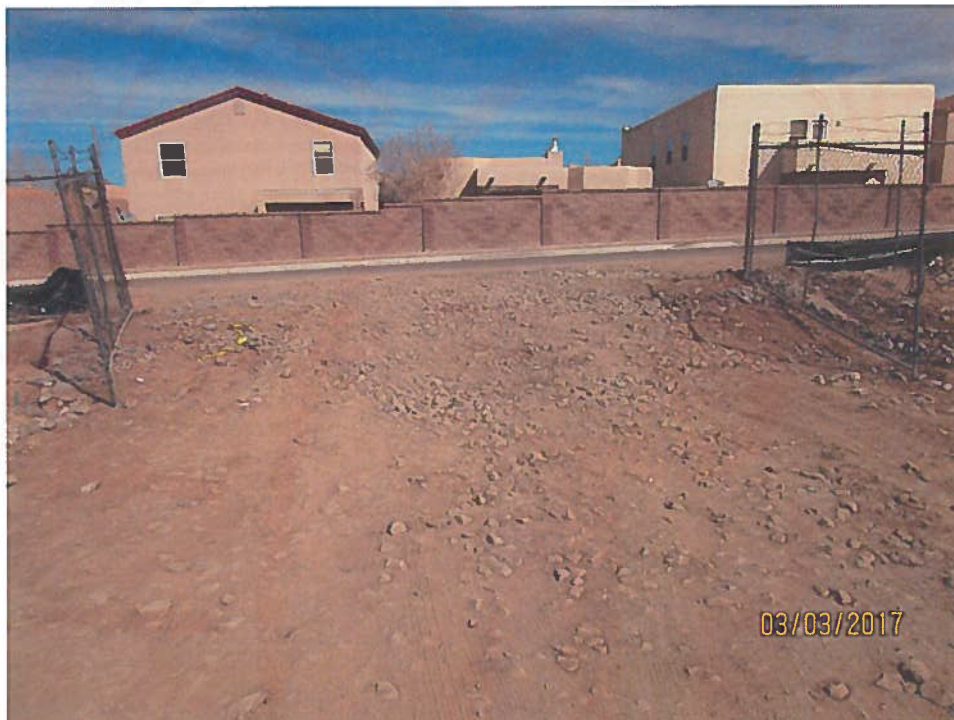
Track-out pad/stabilized construction entrance in poor condition.
