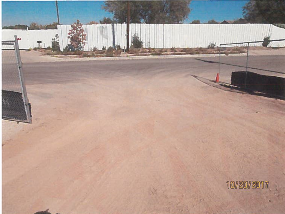
No track-out pad onto Oakland Ave. Sediment in street.
