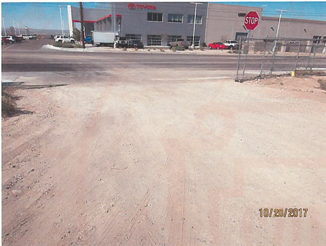
No track-out pad onto San Pedro Blvd. Sediment in street.
