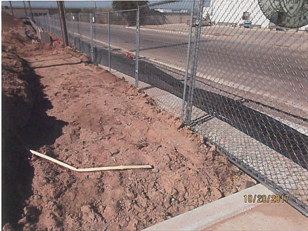
Silt fence not buried.
