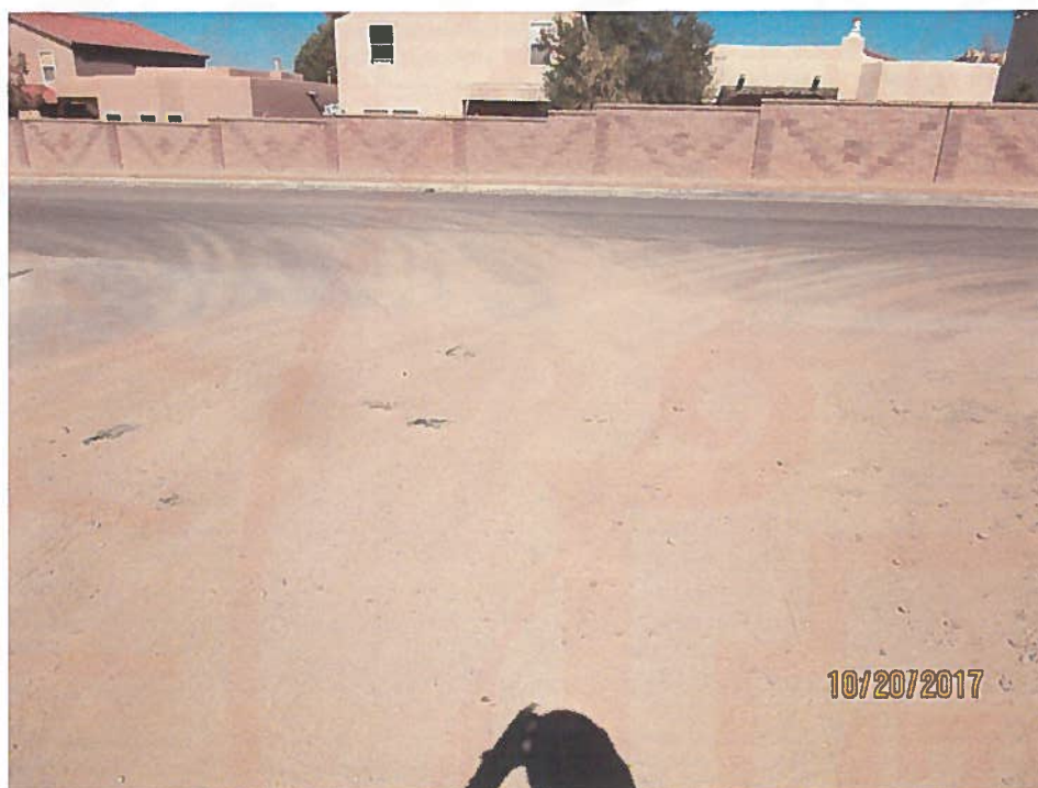
Additional entrance onto Oakland Ave. without a track-out pad. Sediment in street.
