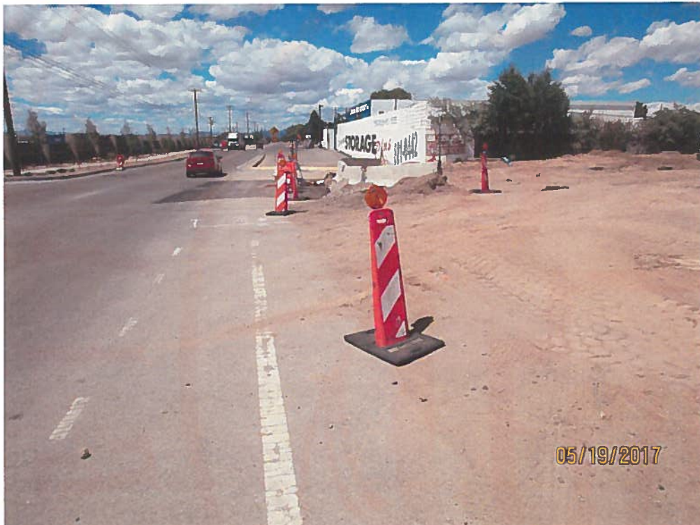
Sediment BMP not installed.
