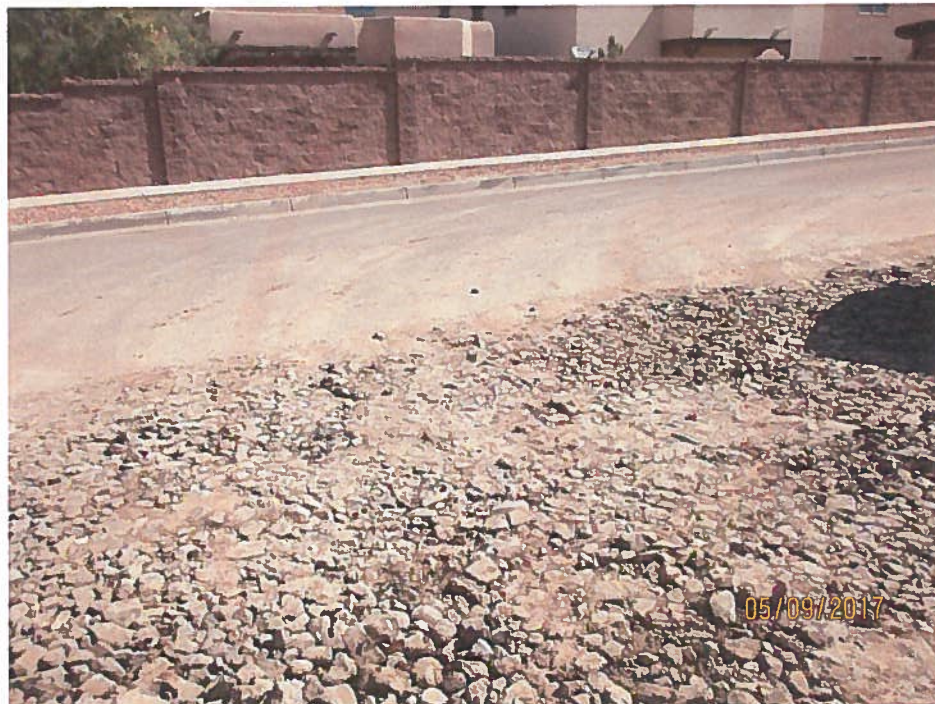
Track-out pad requires maintenance.
