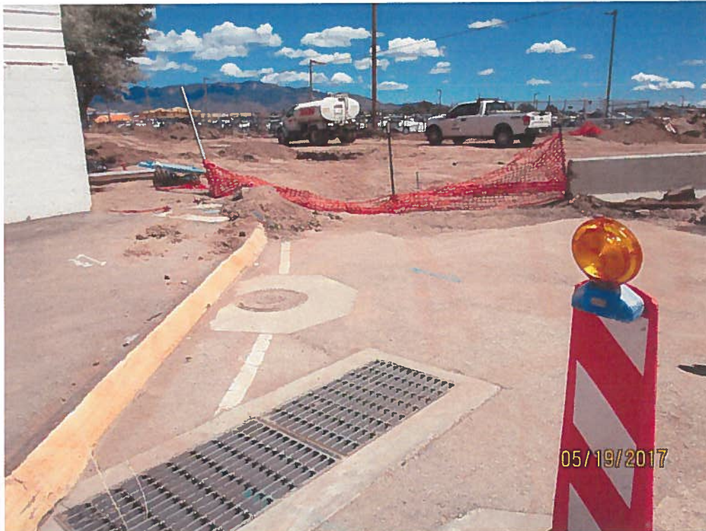
Inlet with no protection and sediment BMP not installed.
