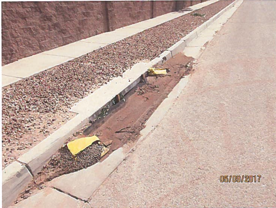
Inlet protection on Oakland requires maintenance.
