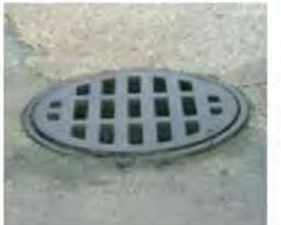
1. Remove sediment, debris, ice and snow from the inlet grate surface and surrounding area.
