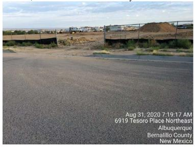
3. West construction entrance missing and has had trackout for 7 days
