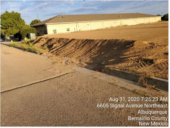
4. Silt fence missing on west half of site
