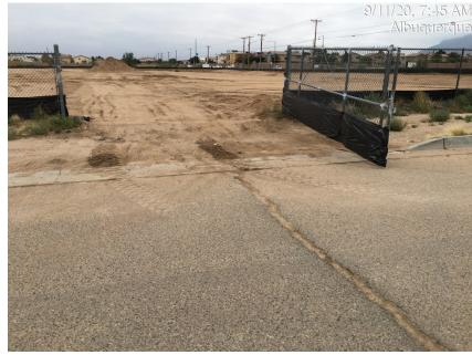
3. West construction entrance missing and has sediment in the street a couple hundred feet downstream in Signal Ave.
