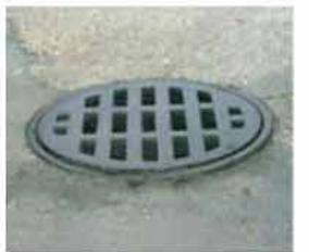
Remove sediment, debris, ice and snow from the inlet grate surface and surrounding area.
