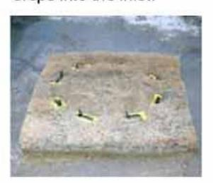
3. Position the mat. Place Inlet Filter on grate with the net side down, flush to the back edge and extending beyond the grate opening on the front and both sides. The zip ties attach Inlet Filter to the inlet grate cover WITHOUT LIFTING THE GRATE COVER.
