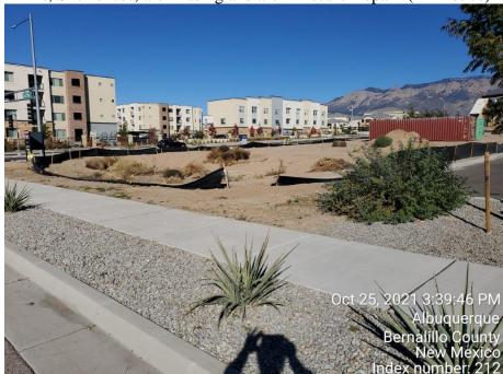
4. BMPs, Silt Fences, are missing and are in need of repair. (2<sup>nd</sup> Notice)
