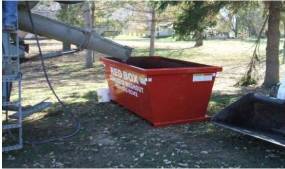
Concrete washout service
