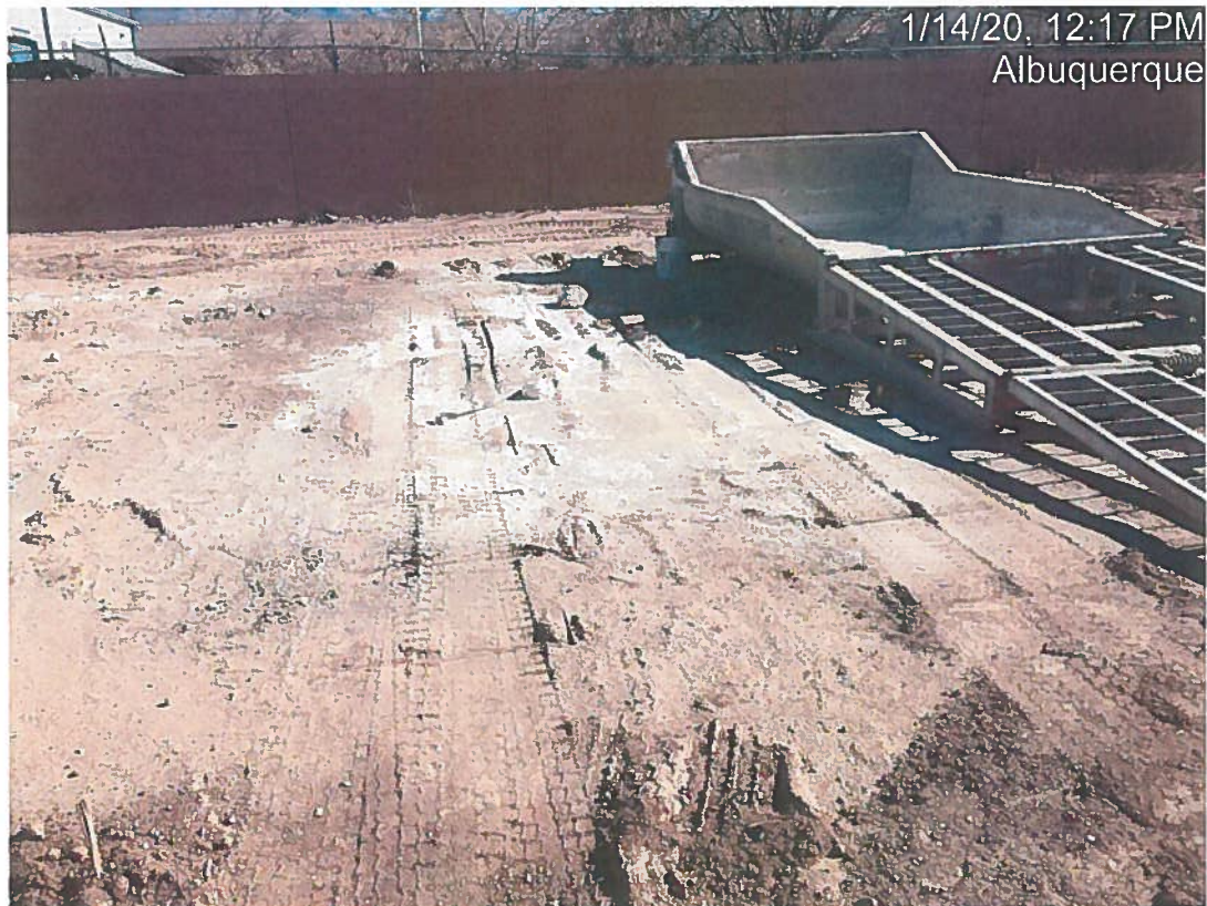
Washout not in acceptable container.
