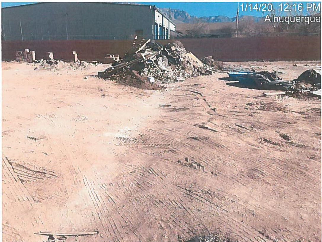
Cutback BMP missing and track-out
