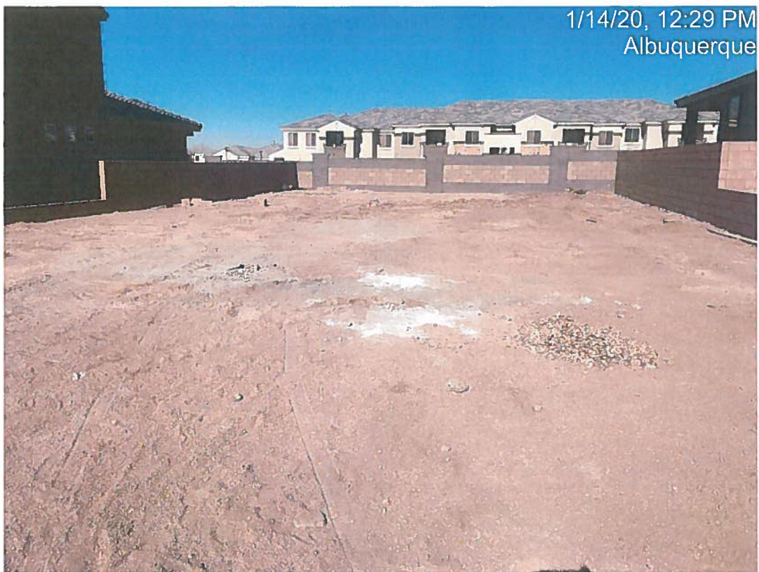
Washout not in acceptable container.
