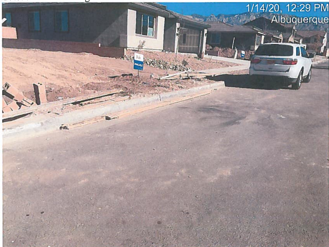
Cutback BMP missing and track-out
