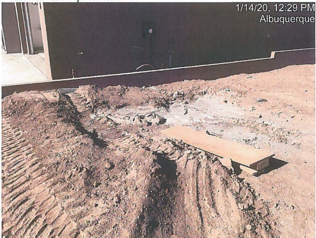
Washout not in acceptable container.
