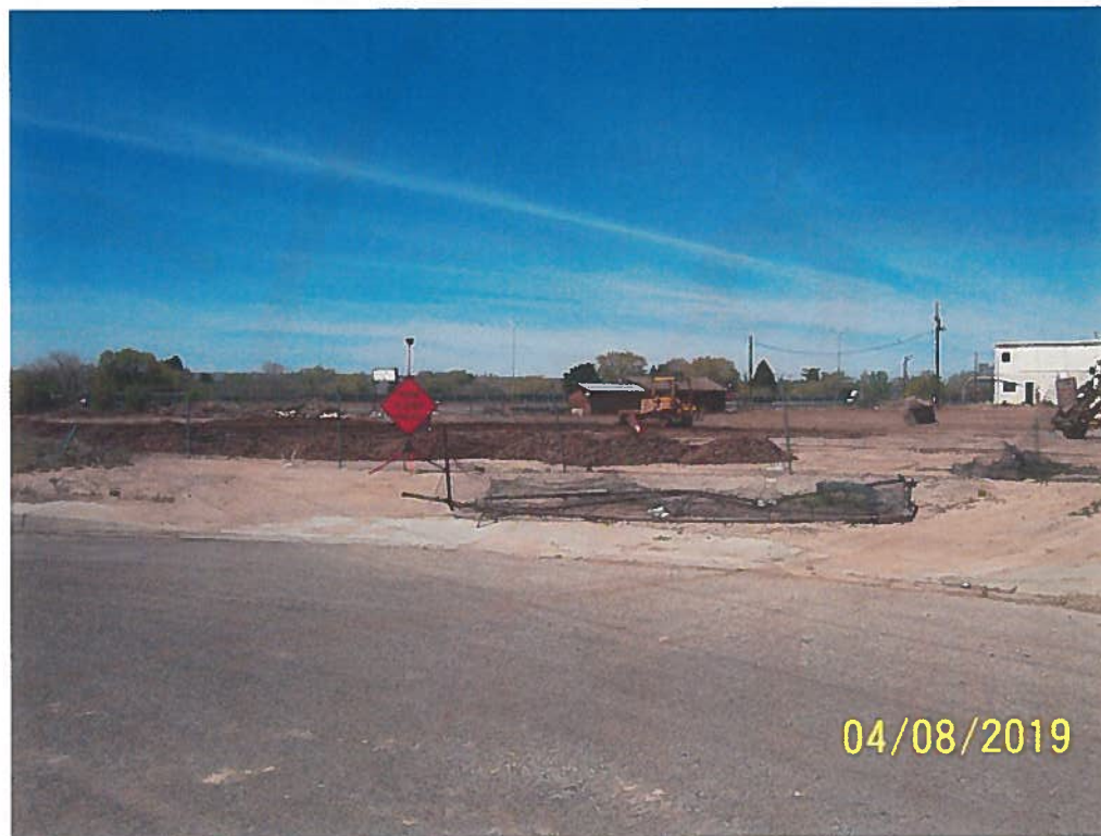
Earth disturbed at site. No sediment BMPs.
