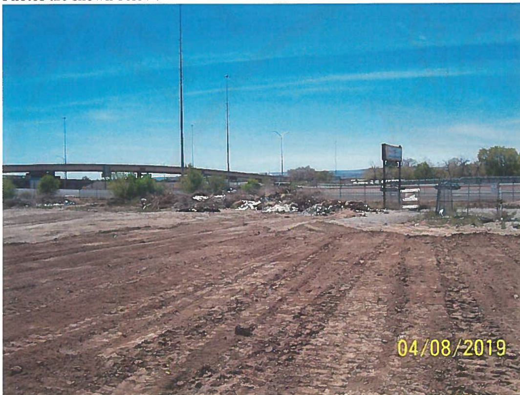
Earth disturbed at site. No sediment BMPs.
