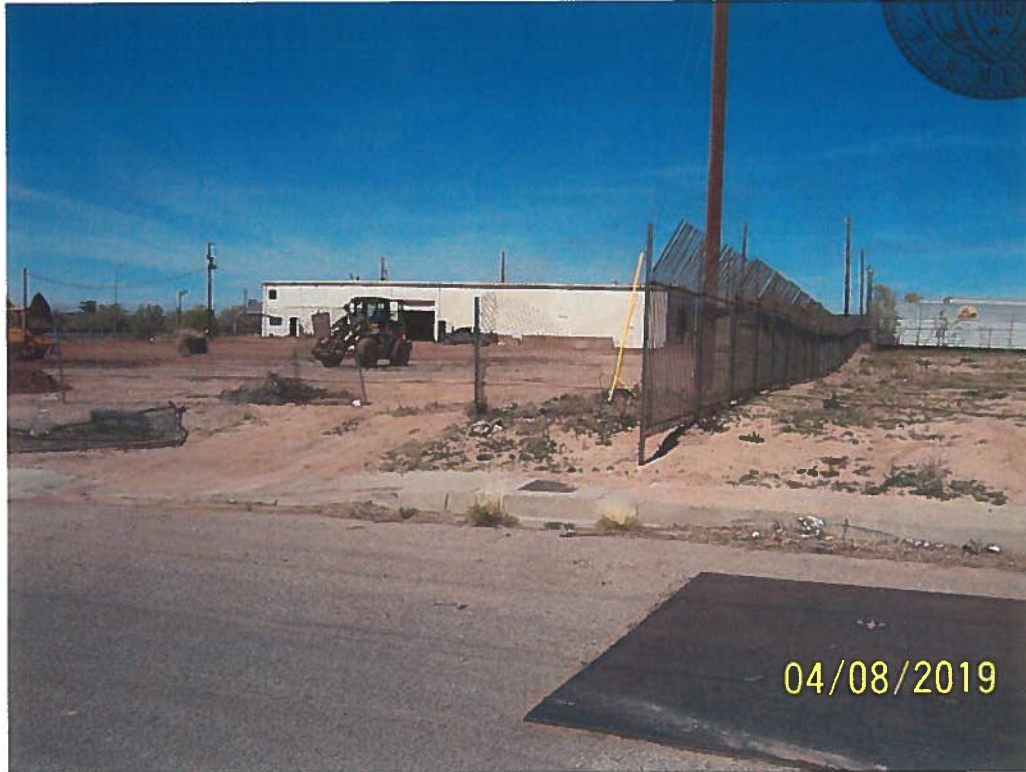
Earth disturbed at site. No sediment BMPs.
