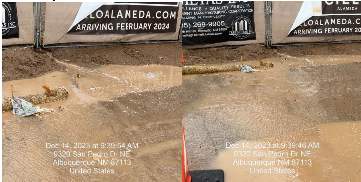
2 Erosion and undercut of BMPs with discharge on San Pedro Dr.
