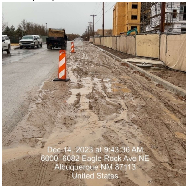
1 Tracks through exposed soil and track-out on Eagle Rock Ave.
