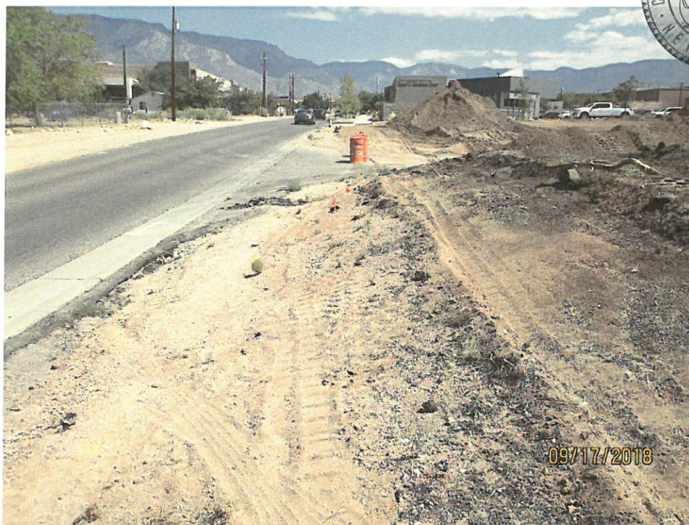
No Stormwater Controls along Holly Ave.
