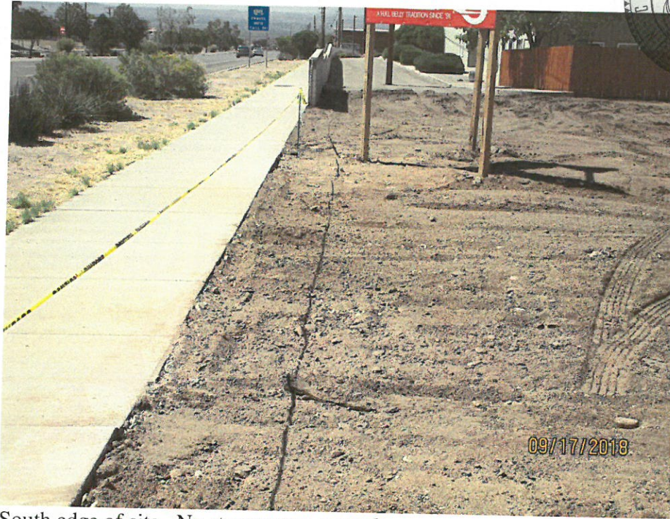
South edge of site. No stormwater controls.
