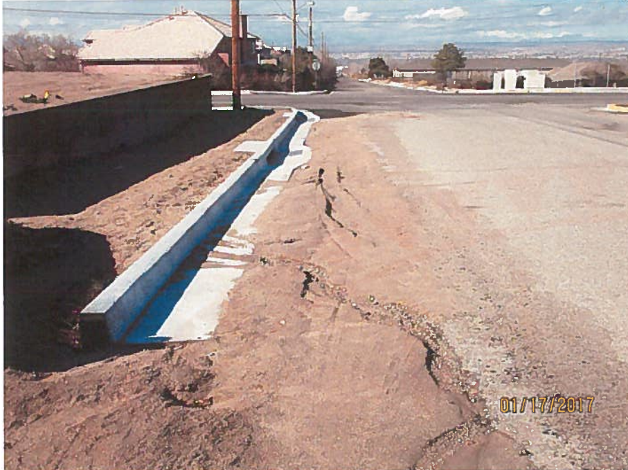
No inlet protection and sediment in gutter.
