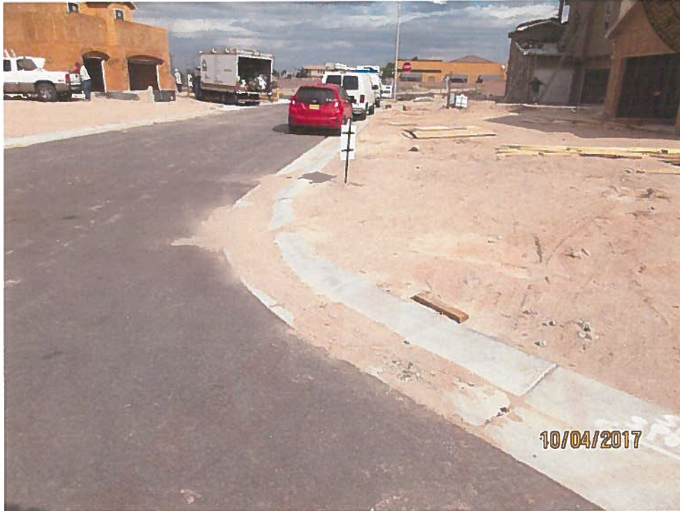
No sediment BMP. Sediment in street.
