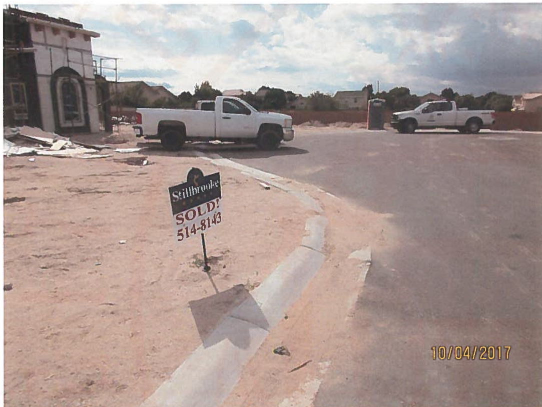
No sediment BMP. Sediment in street.
