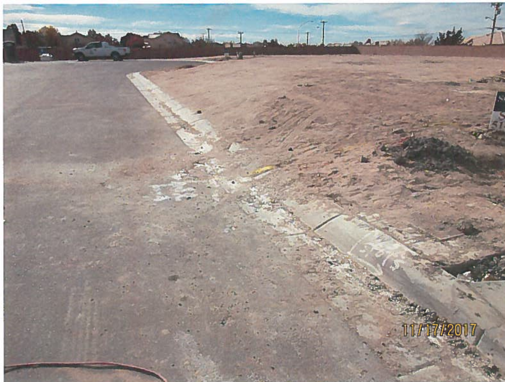
Wash-out in gutter pan.
