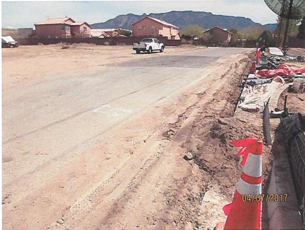
Too much loose dirt on the south side of Signal without a sediment BMP.
