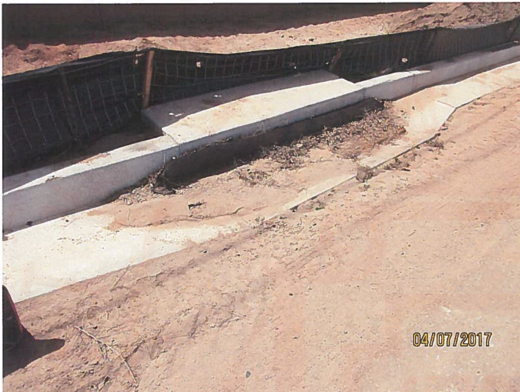
Inlet protection requires maintenance.
