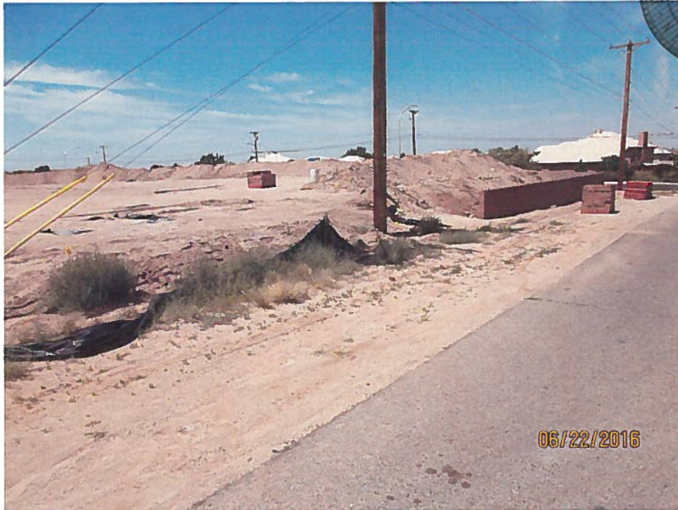
Partial silt fence installation and silt fence requires maintenance on Signal Rd West of the construction entrance.
