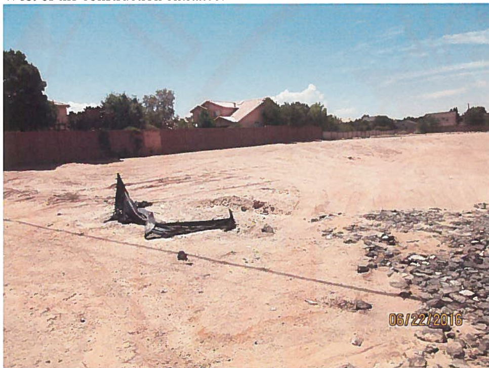
Partial silt fence installation and silt fence requires maintenance on Signal Rd East of the construction entrance.
