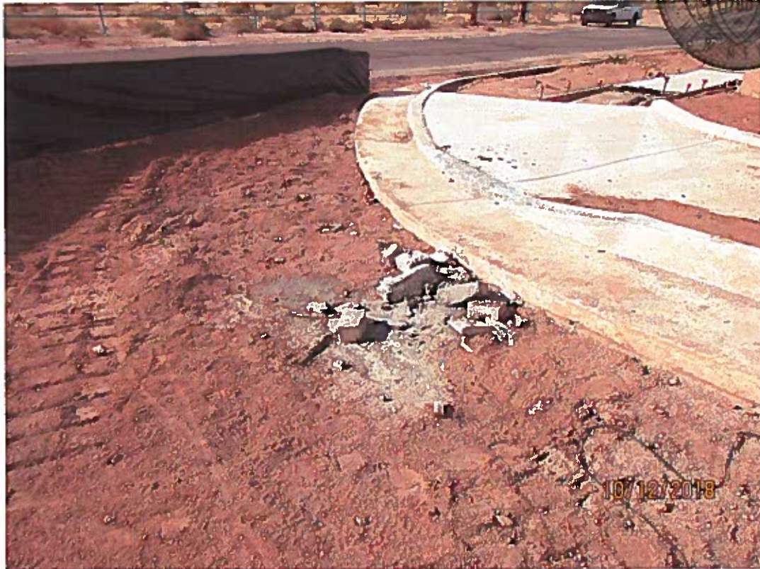
Concrete wash-out.
