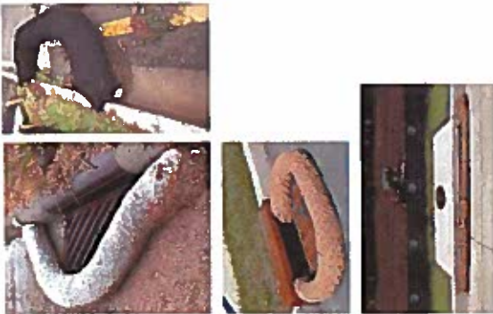
Curb Storm Inlet Protection with Traps
