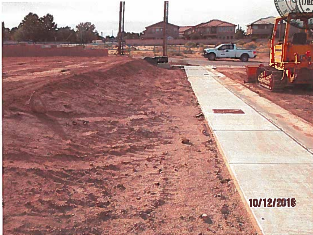
No sediment BMP for graded lots.
