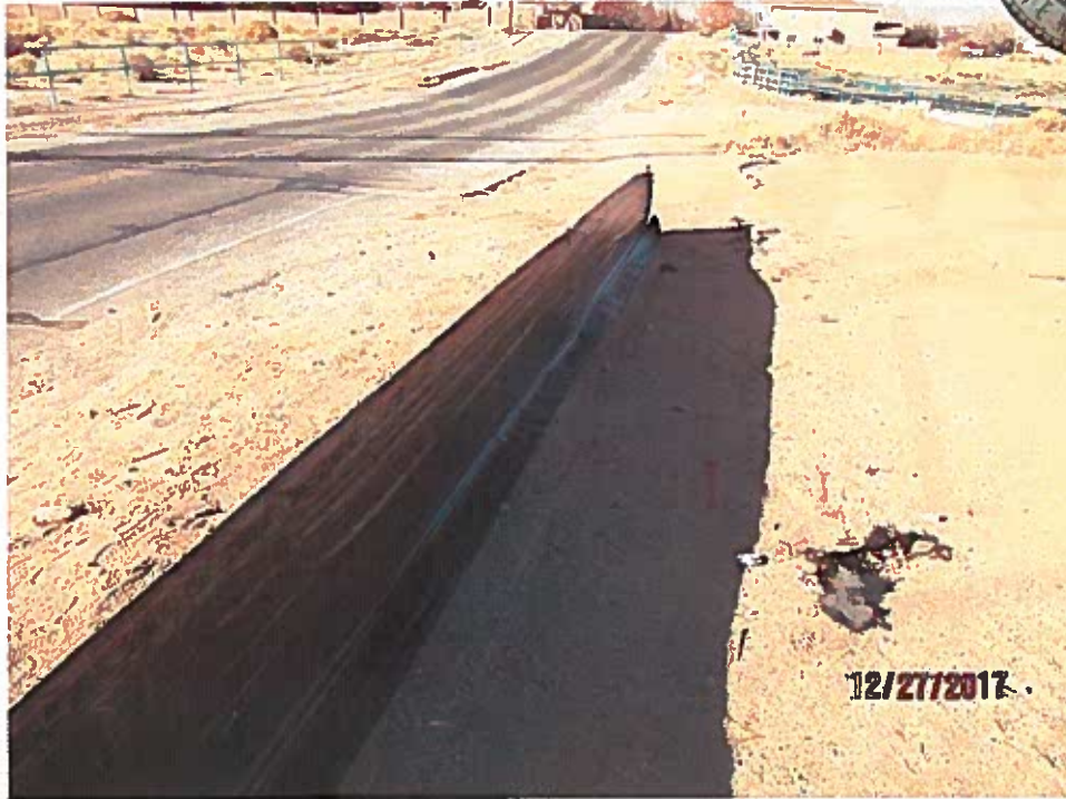
Silt fence is not buried.
