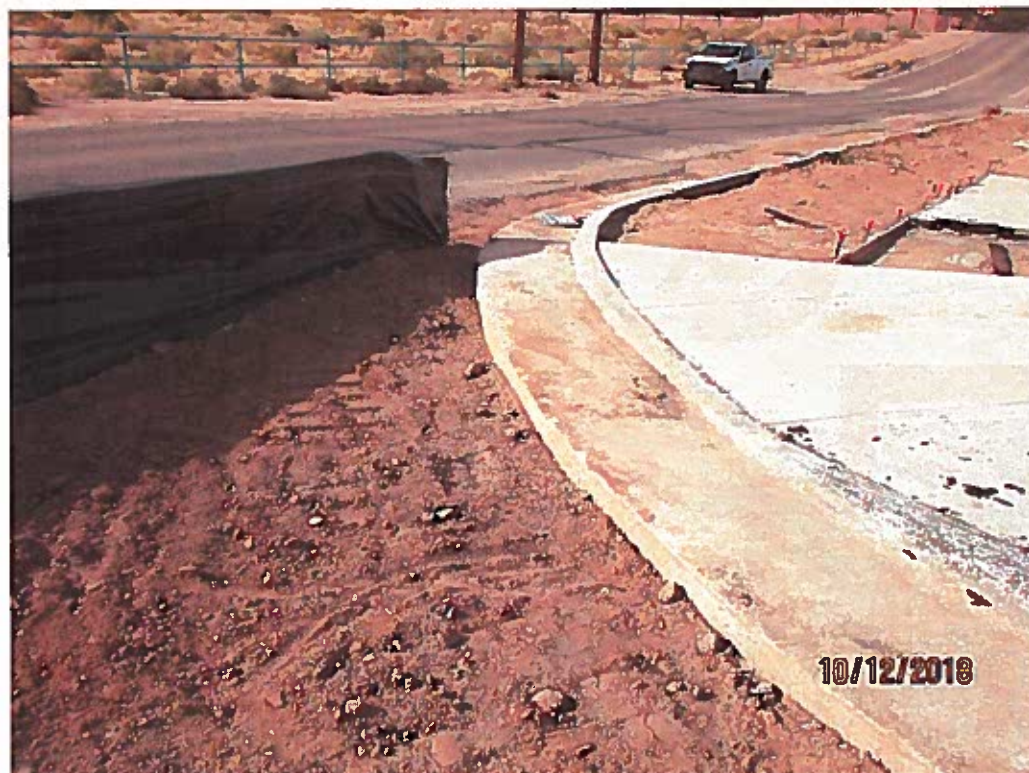
Wyoming south end- No sediment BMP for gutter and gap next to gutter.
