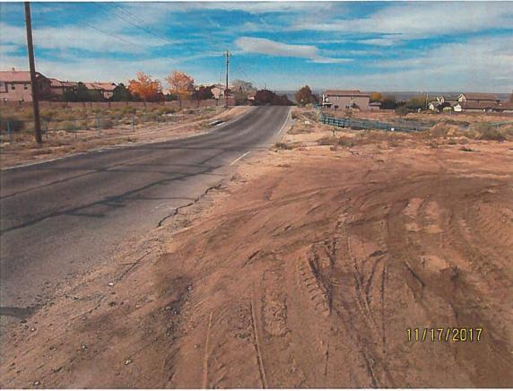
No stabilized Construction Entrance to site and no silt fence along street.
