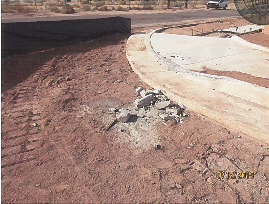
Concrete wash-out.
