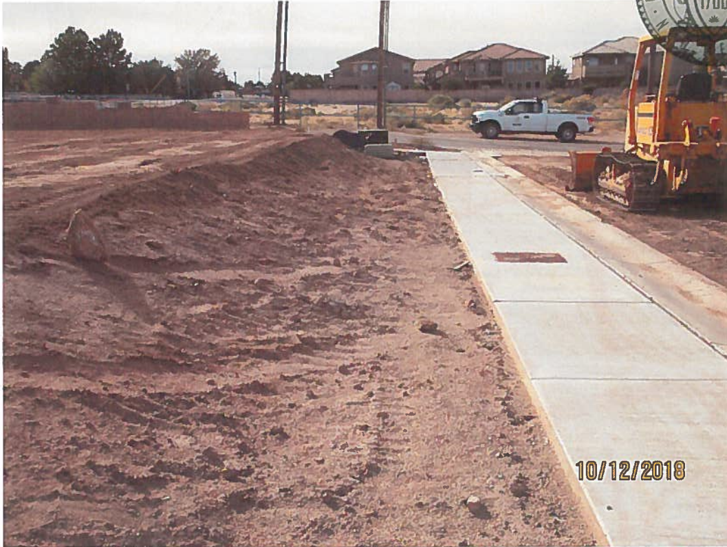
No sediment BMP for graded lots.
