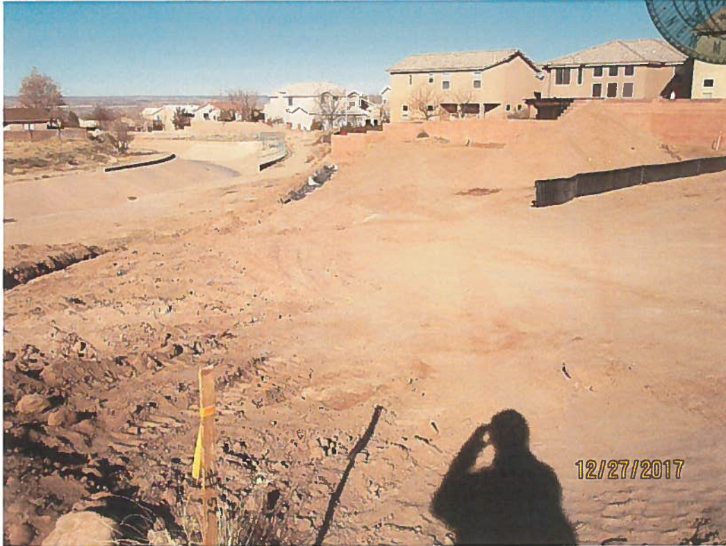
Silt fence does not extend across western edge of disturbed area.
