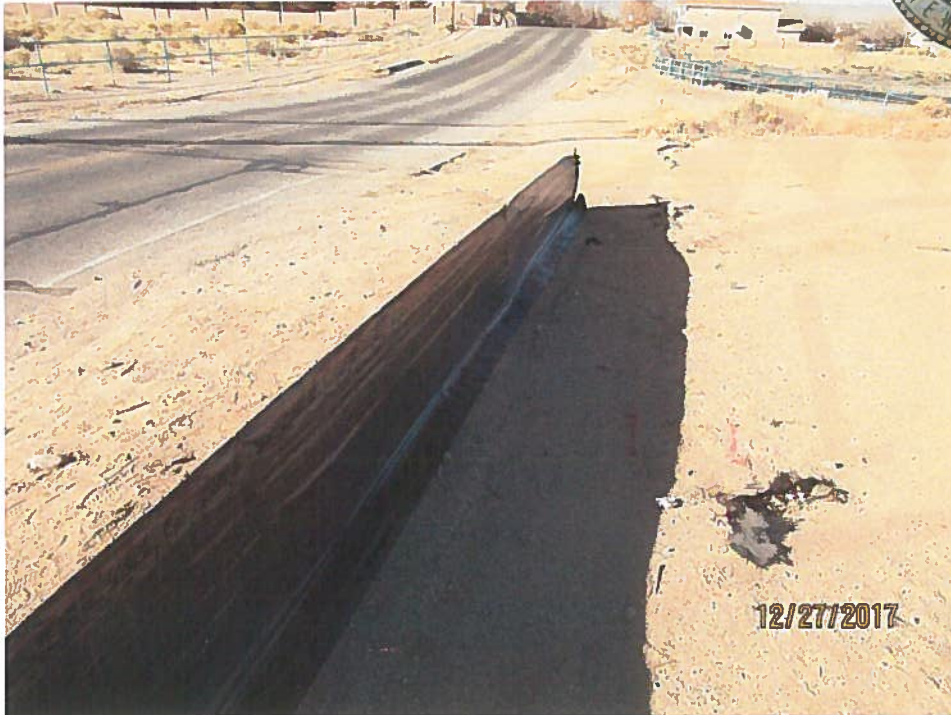
Silt fence is not buried.
