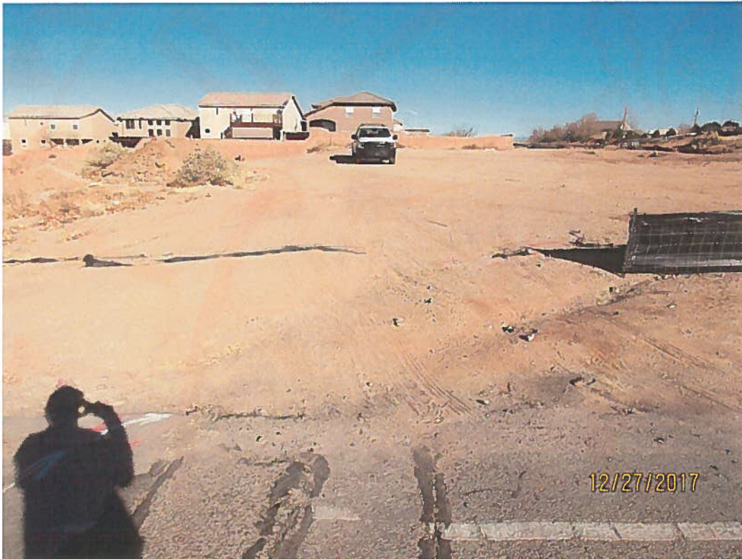
No stabilized Construction Entrance/track-out pad.
