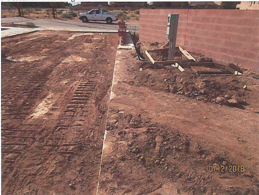
West gutter-No sediment BMP.
