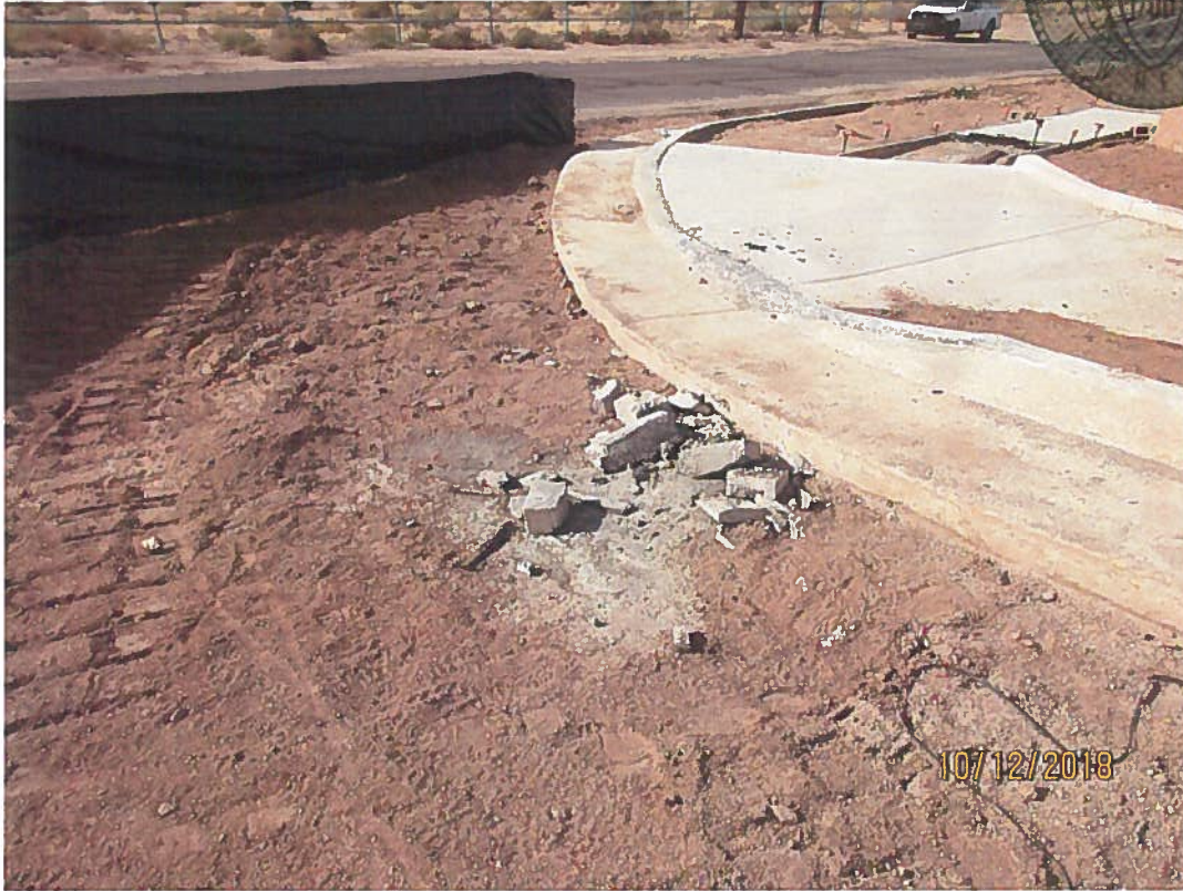
Concrete wash-out.
