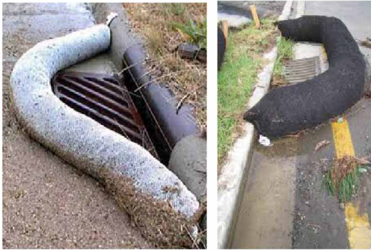
Curb Storm Inlet Protection with Wattles
