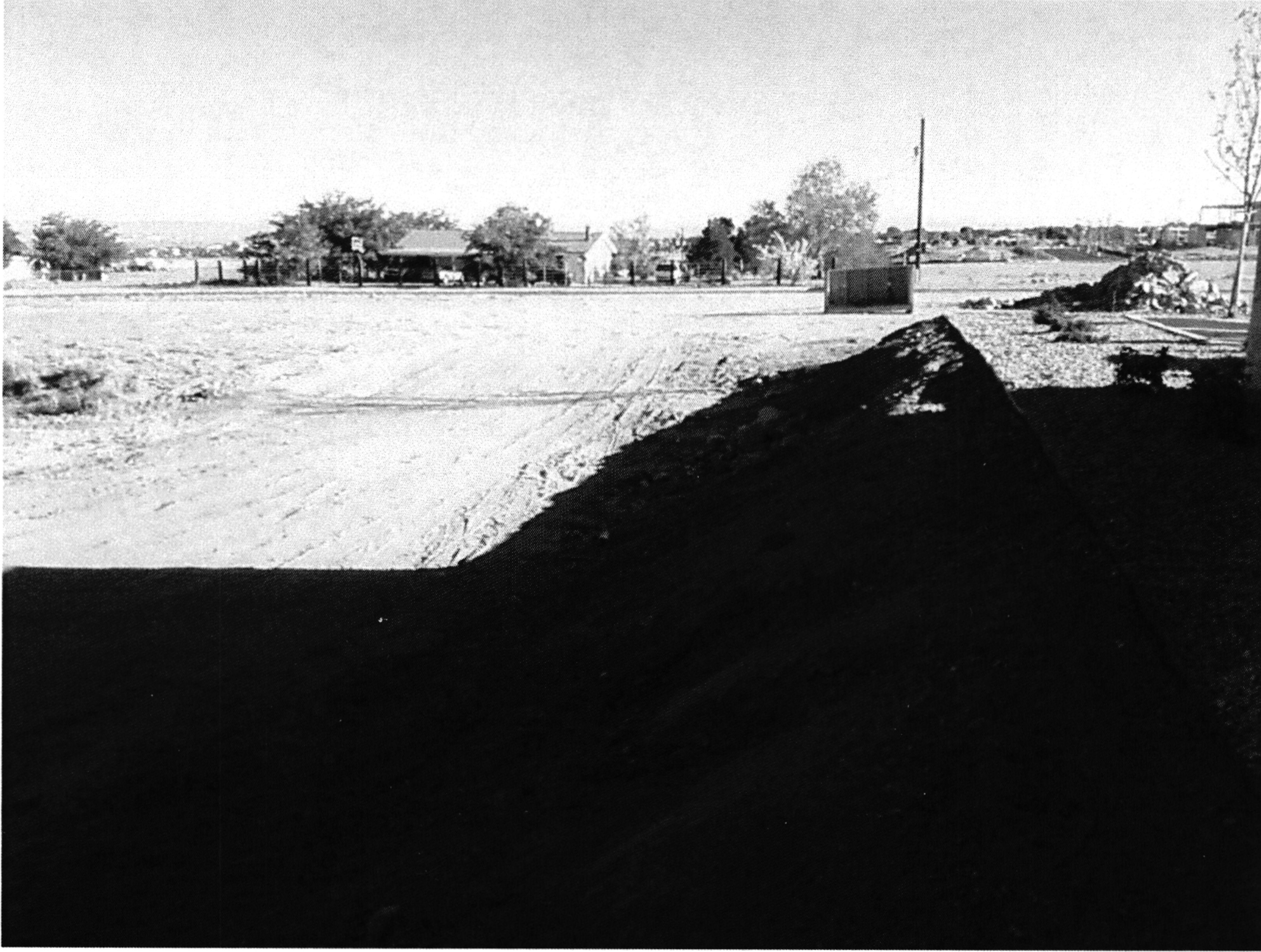
Slope west of parking lot. Sections steeper than 3:1.
