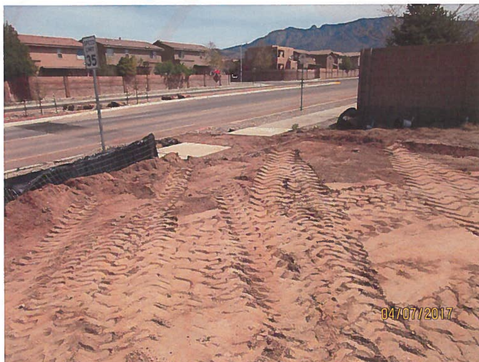
Gap in silt fence northeast corner.
