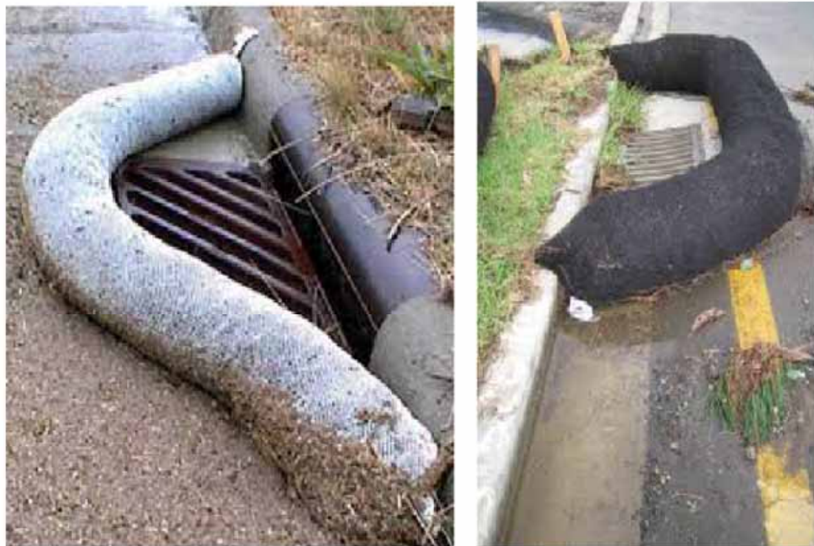
Curb Storm Inlet Protection with Wattles
