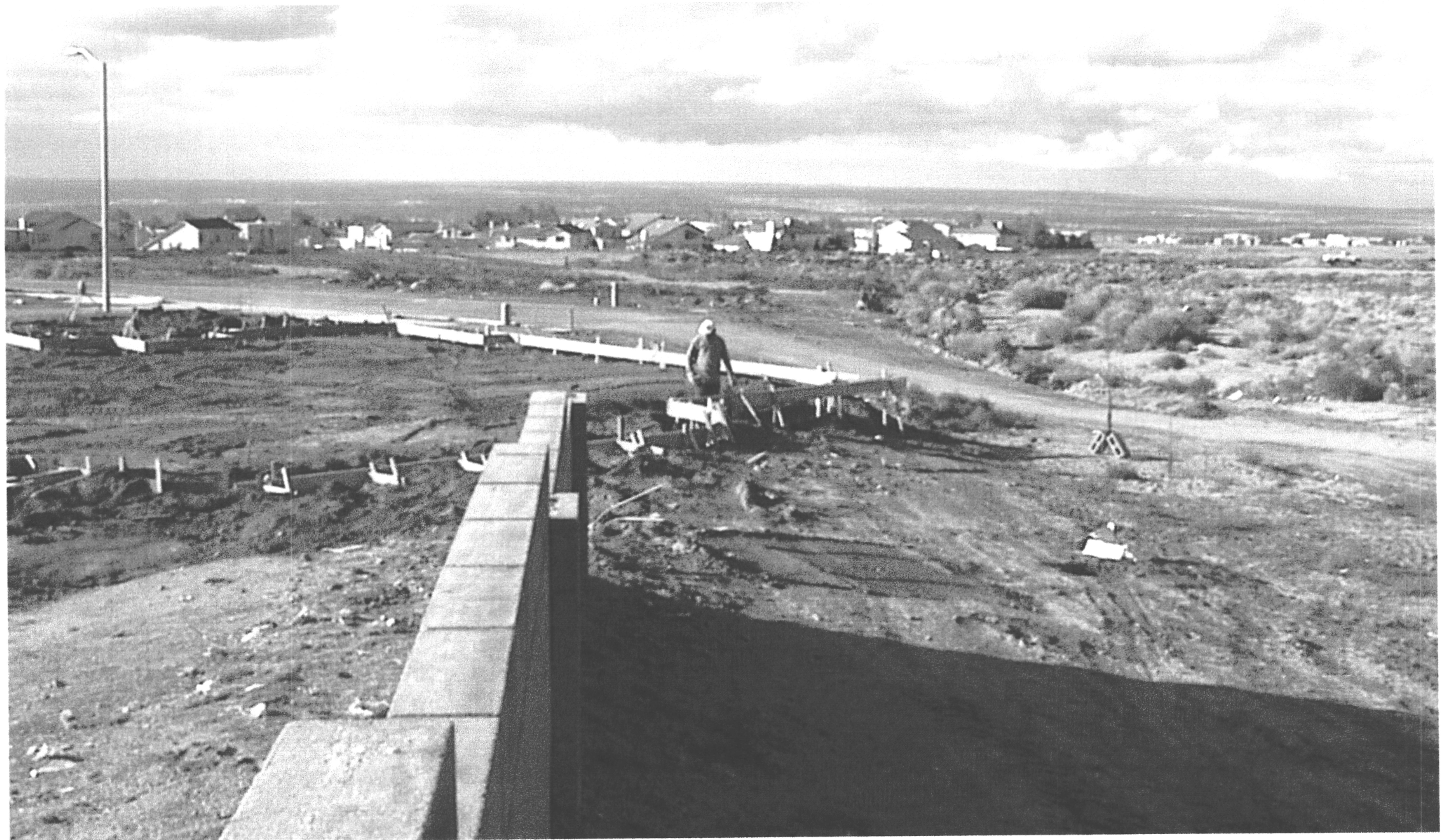
Lot 6 looking northwest. Notice construction extending beyond floodwall, geeting close to apparent arroyo flowpath. ?Is this per approved plan? ?Per properly approved plan?
