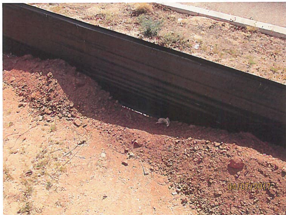
Silt fence not buried.
