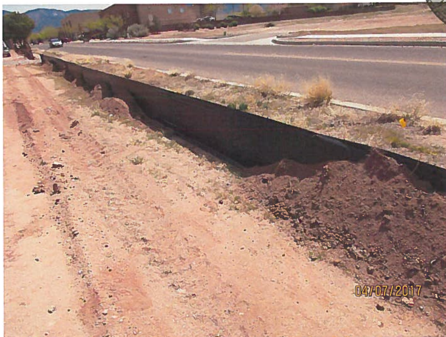
Dirt piled against silt fence sporadically.
