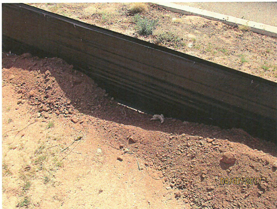
Silt fence not buried.
