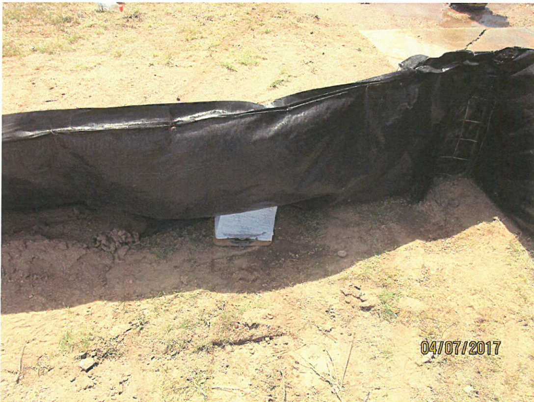
Silt fence not buried at outfall location in southwest corner.
