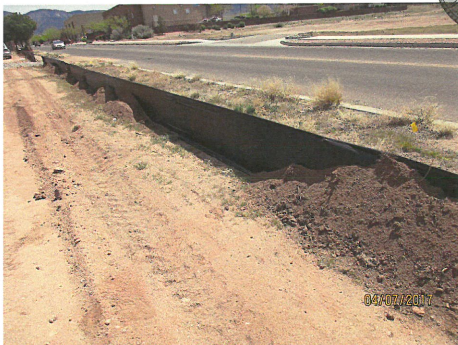
Dirt piled against silt fence sporadically.
