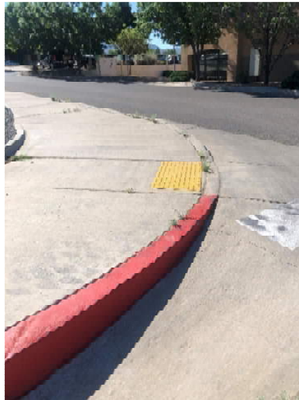
Truncated Domes installed on four ramps in right-of-way
