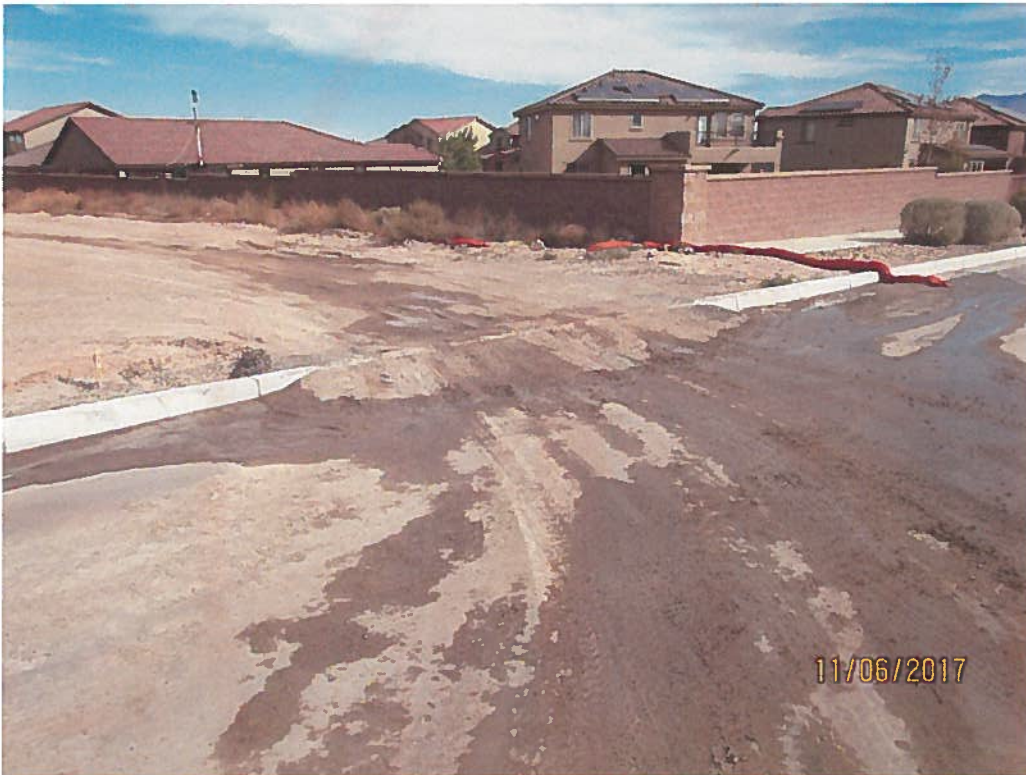
Require track-out pad at water truck haul road entrance onto Vista Vieja Ave.
