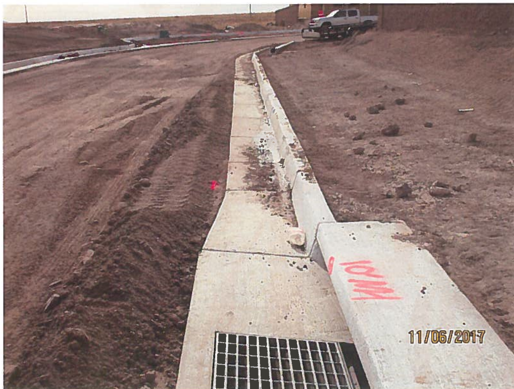
Sediment and trash in gutter. No inlet protection.
