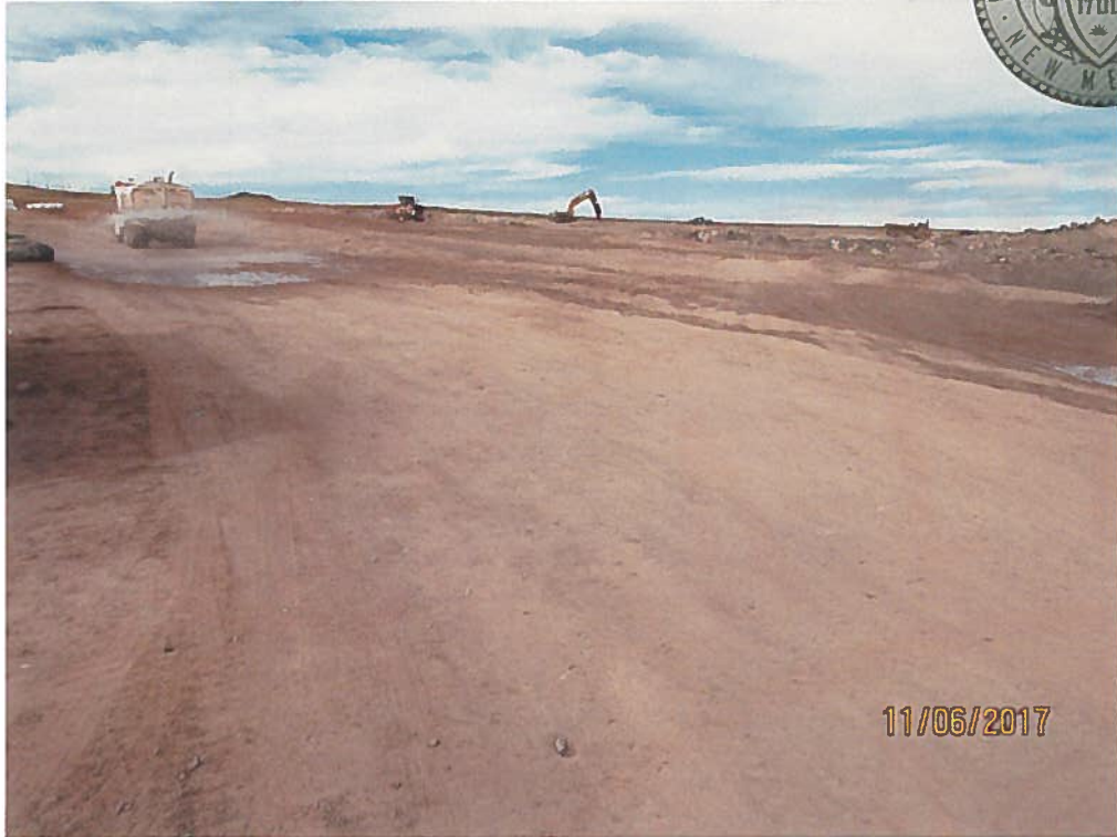
No erosion or sediment BMP-west area.
