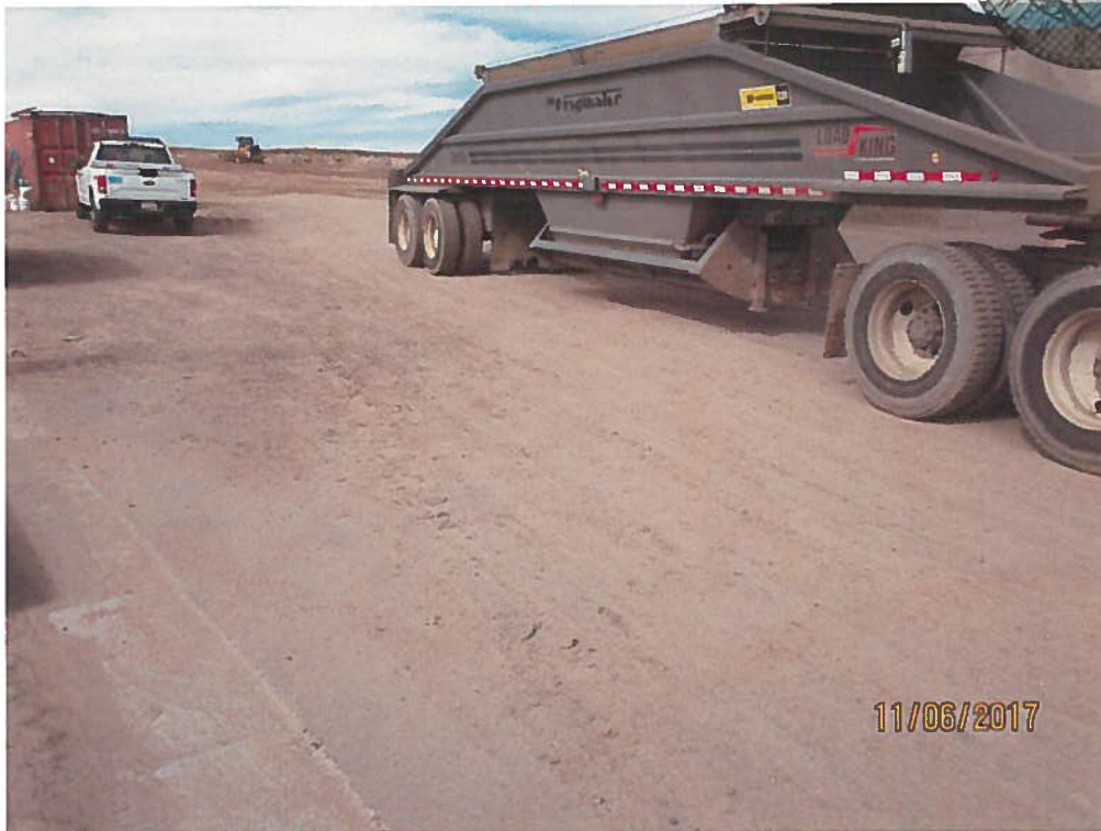
No track-out pad from west dirt area onto Vista Vieja Ave.
