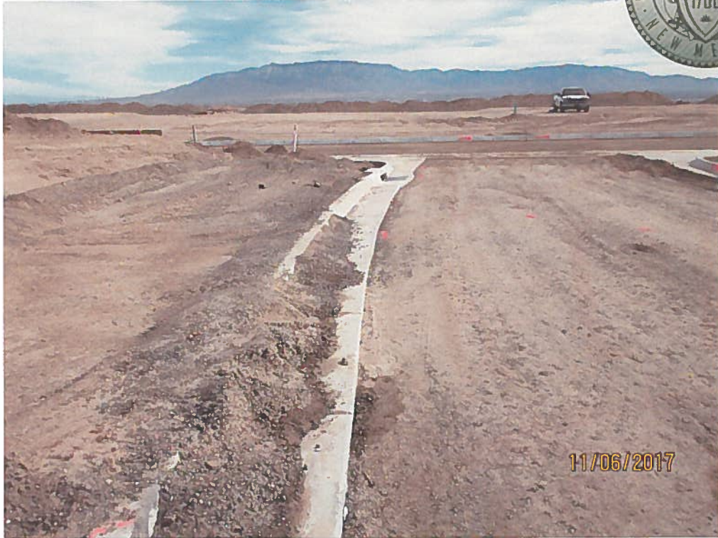
Sediment in gutter. No inlet protection. Numerous locations.
