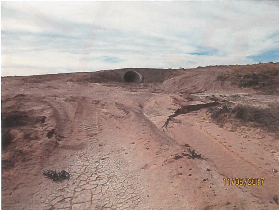
Storm drain outfall with no erosion protection.
