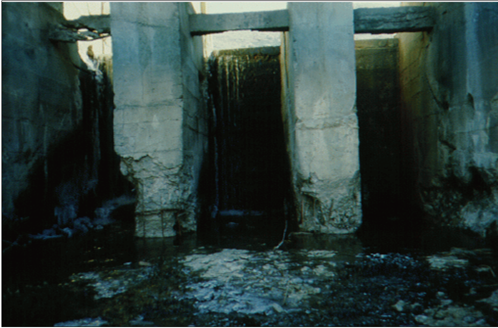
Figure 1.—Lack of maintenance has resulted in near loss of this irrigation structure.
