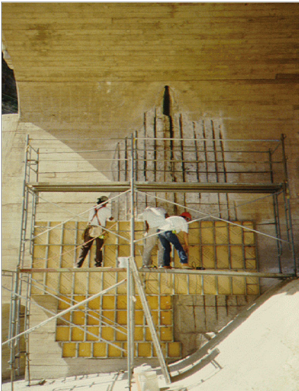
Figure 55.—If forms are required for epoxy-bonded concrete repairs, they should be installed at least once prior to application of the epoxy bond coat to ensure that they fit as planned and that they can be installed and filled before the bond coat hardens.
