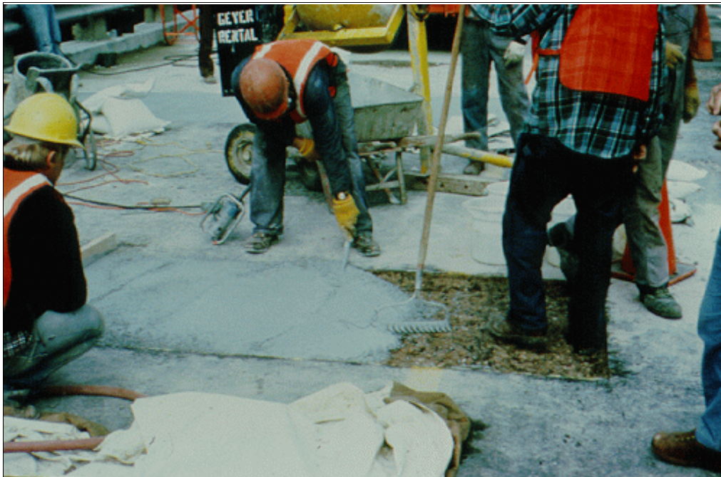
Figure 58.—Small stinger vibrators can be used to consolidate shallow depths of polymer concrete.
