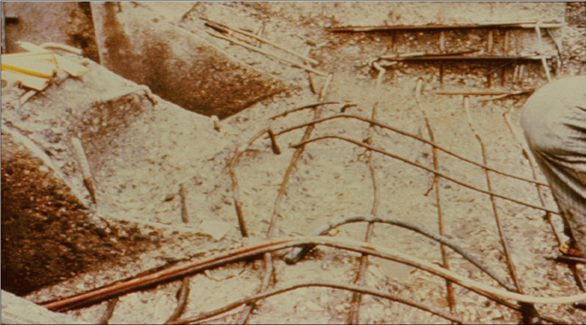
Figure 23.—Abrasion-erosion damage in a concrete stilling basin.
