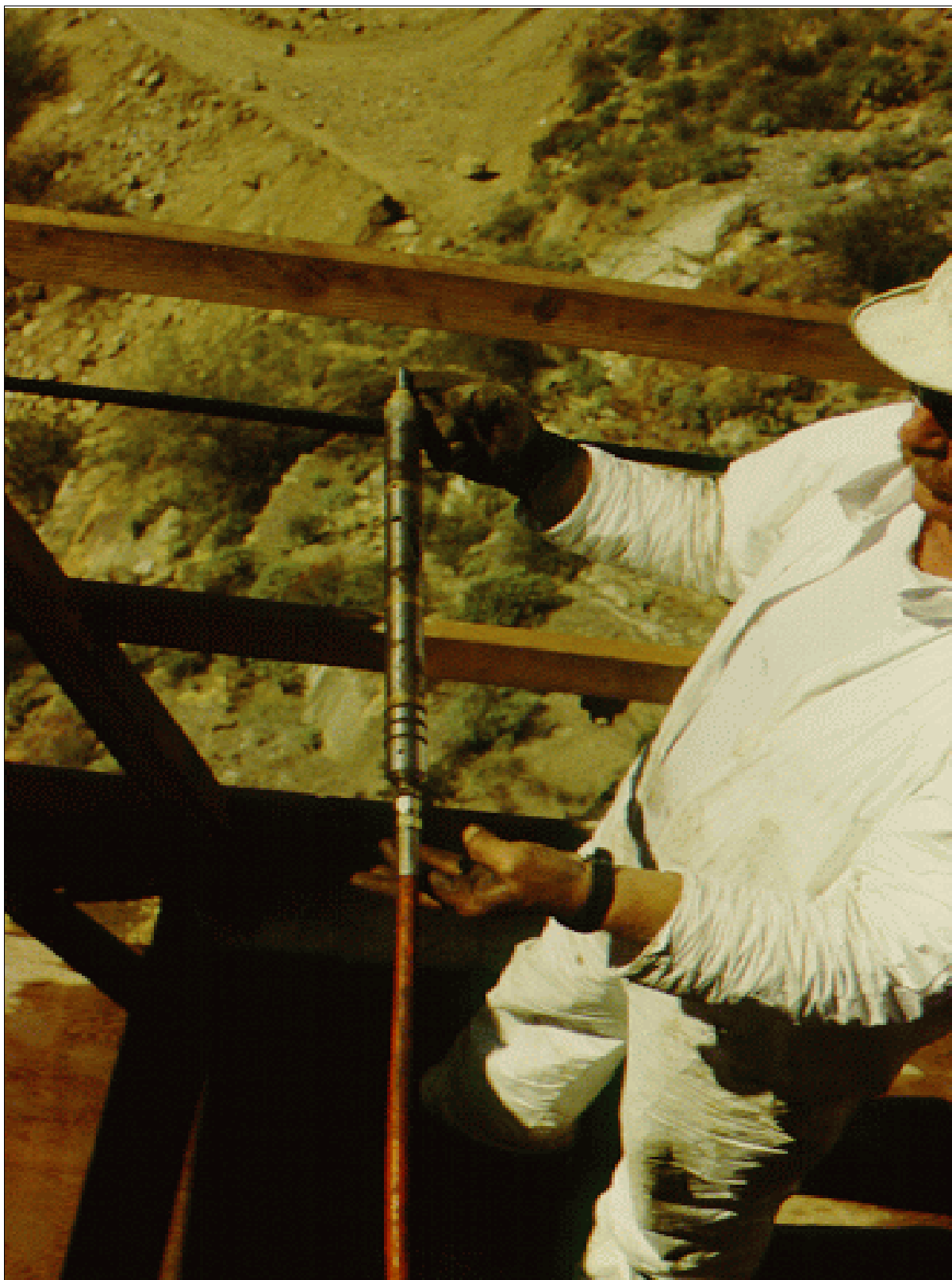
Figure 67.—A proprietary downhole packer allows separation of the resin components until they reach the downhole point of injection.
