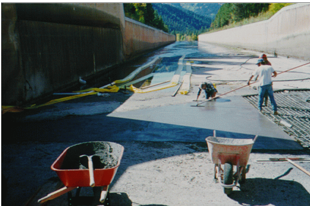
Figure 70.—Using a bull float on a silica fume repair. Finishing must be done immediately after screeding.
