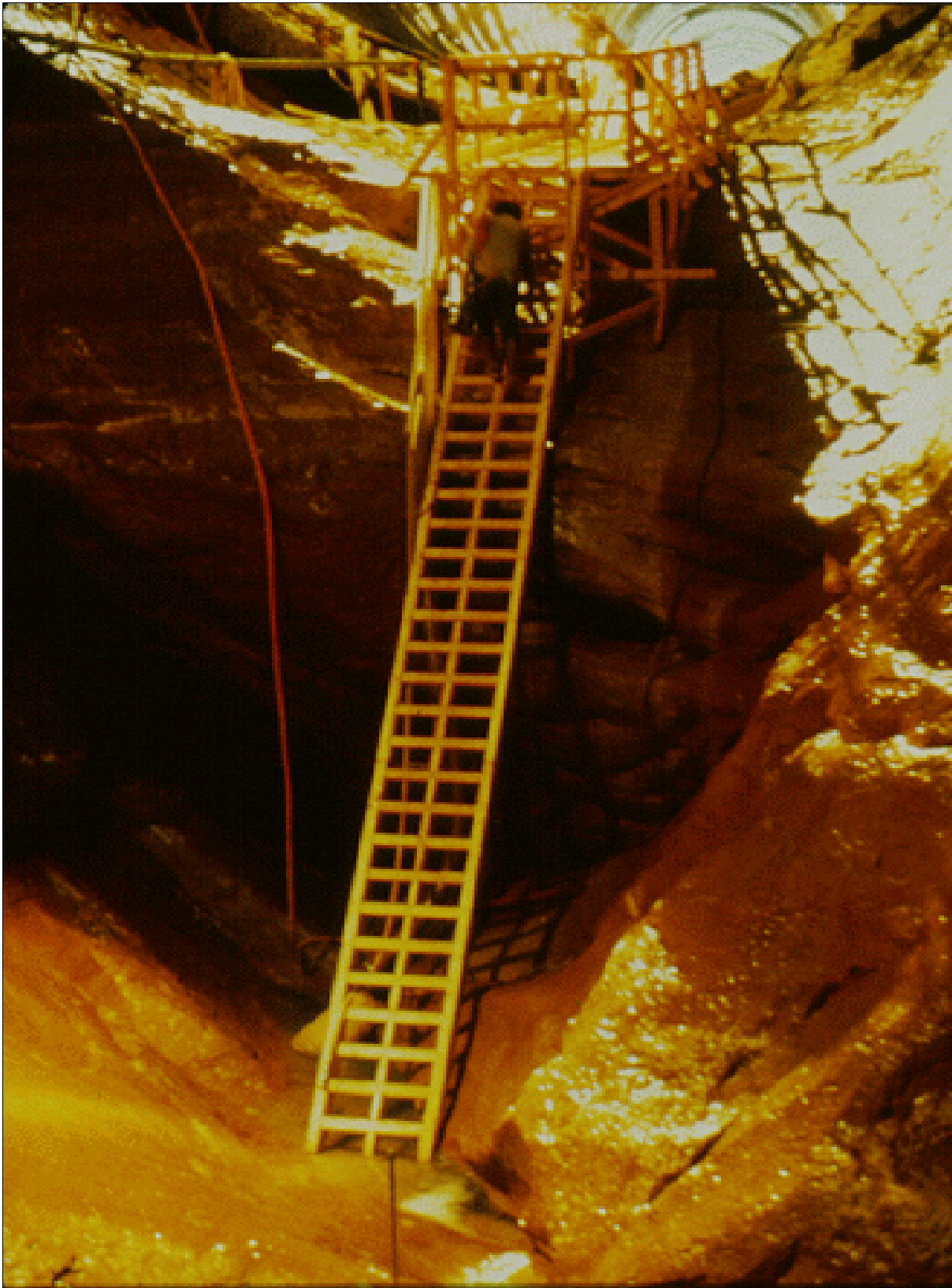
Figure 28.—Extensive cavitation damage to Glen Canyon Dam.
