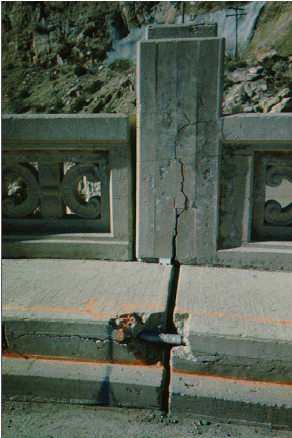
Figure 38.—Multiple causes of damage are apparent in this photograph. Poor design or construction practices placed the electrical conduit too near the surface. A combination of freezing and thawing deterioration and alkali-aggregate reaction is responsible for the cracking and surface spalling on the parapet wall.
