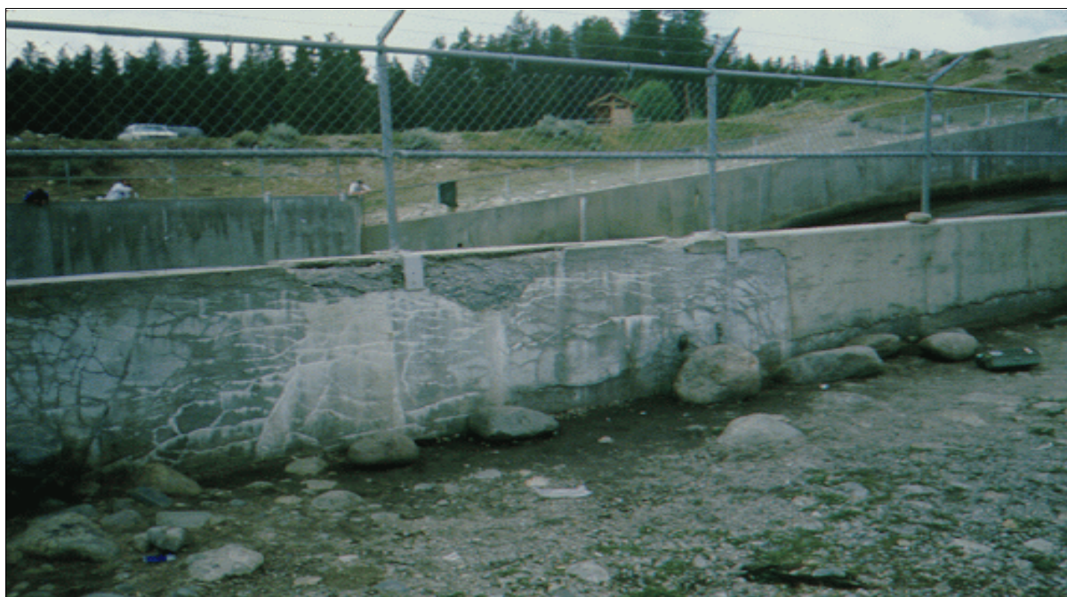
Figure 22.—D-cracking type of freezing and thawing deterioration.
