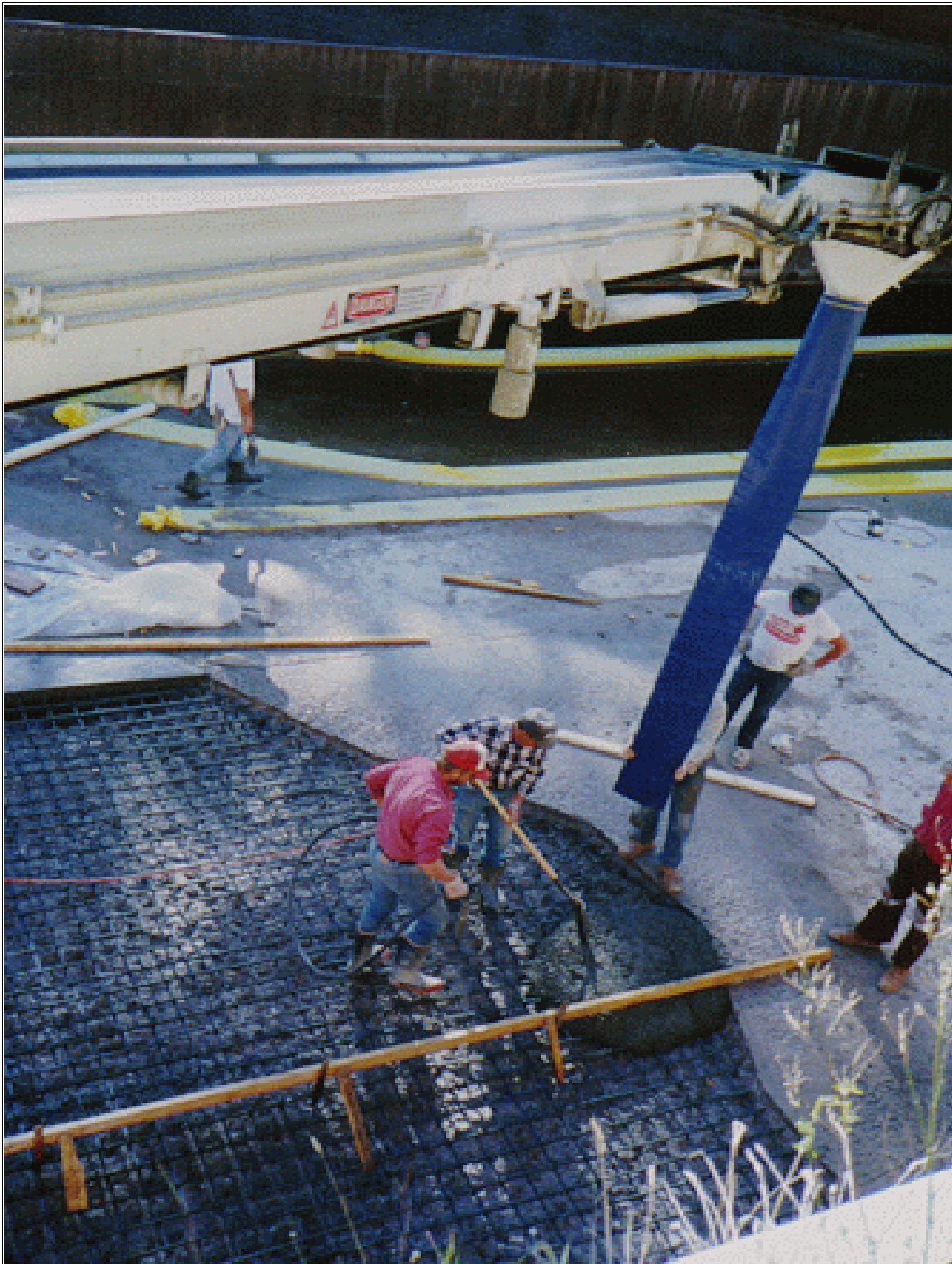
Figure 26.—Placing silica fume concrete to repair a spillway floor damaged by cyclic freezing and thawing and abrasion-erosion.
