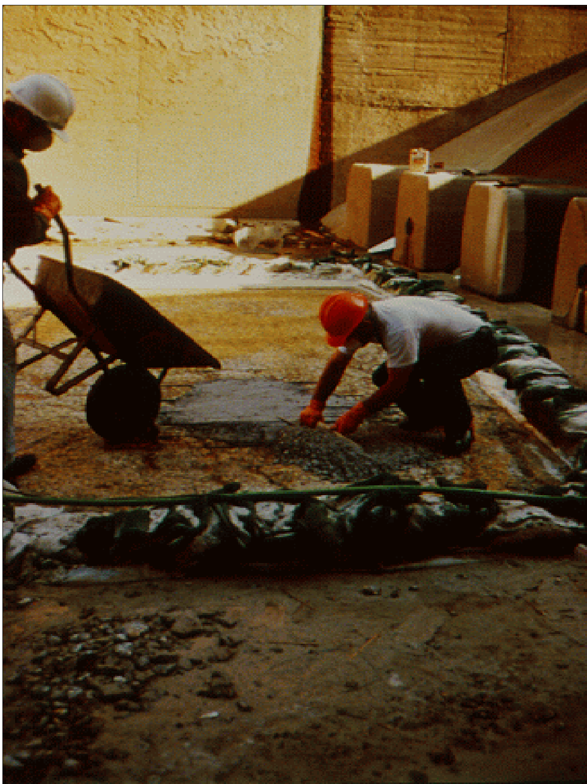
Figure 57.—Placing polymer concrete in a repair area. Sandbags and polyethylene sheeting were used to prevent water from entering the repair area.
