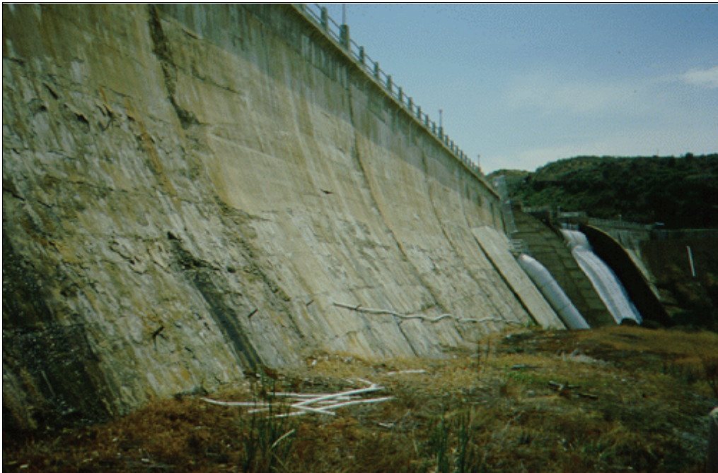
Figure 3.—Freezing and thawing deterioration to the downstream face of this dam does not require repair for safe operation of the structure.
