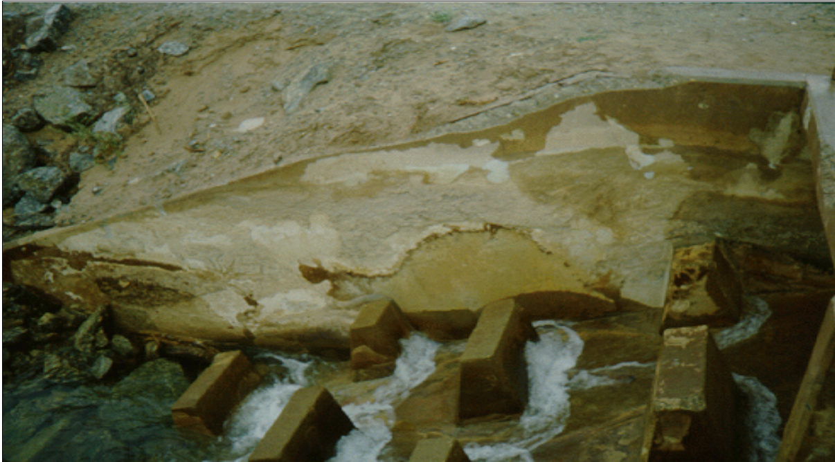
Figure 29.—Concrete damage caused by chloride-induced corrosion of reinforcing steel. The waters contained within this flume had high chloride content.
