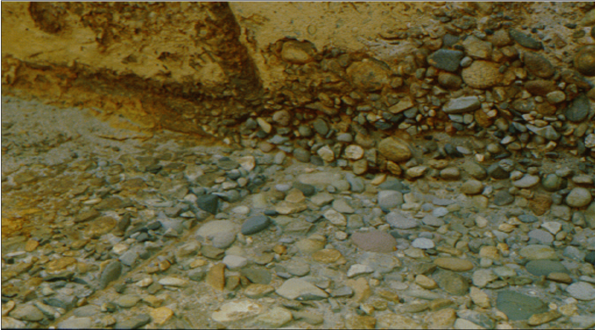
Figure 30.—Concrete deterioration caused by acidic water.
