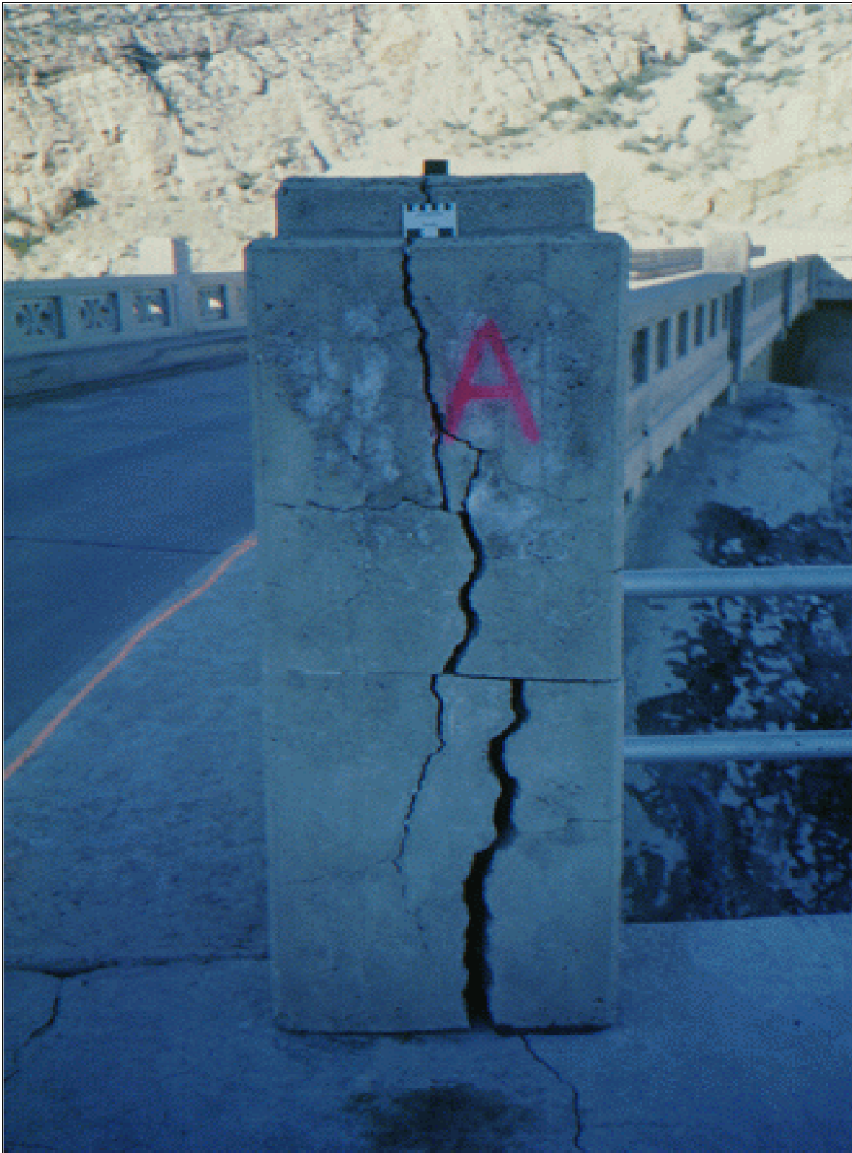
Figure 19.—Severe cracking caused by alkali-aggregate reaction.
