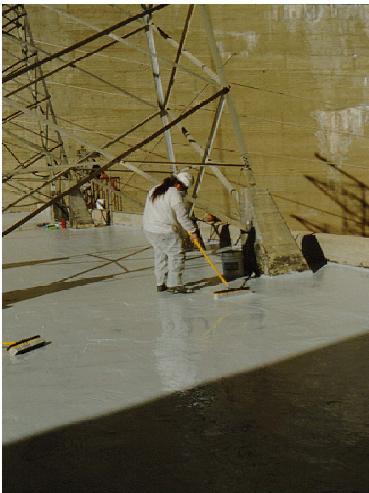
Figure 60.—The thin PC overlay system may be applied with push brooms, squeegees, or heavy industrial grade paint rollers.
