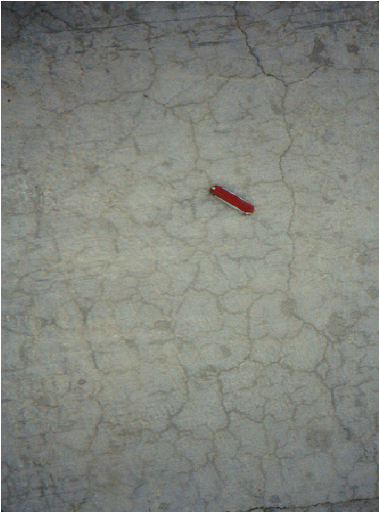
Figure 32.—Typical appearance of drying shrinkage cracking.
