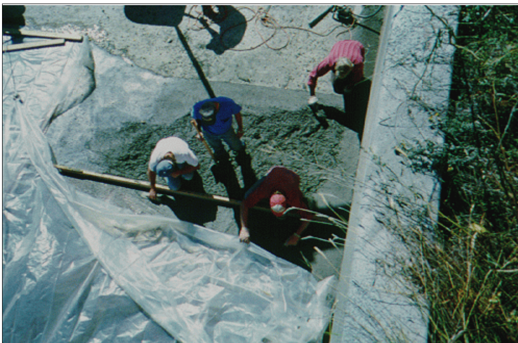
Figure 71.—Curing compound and polyethylene sheeting should be applied to cure silica fumeconcrete as soon as finishing is completed if drying shrinkage cracking is to be prevented.
