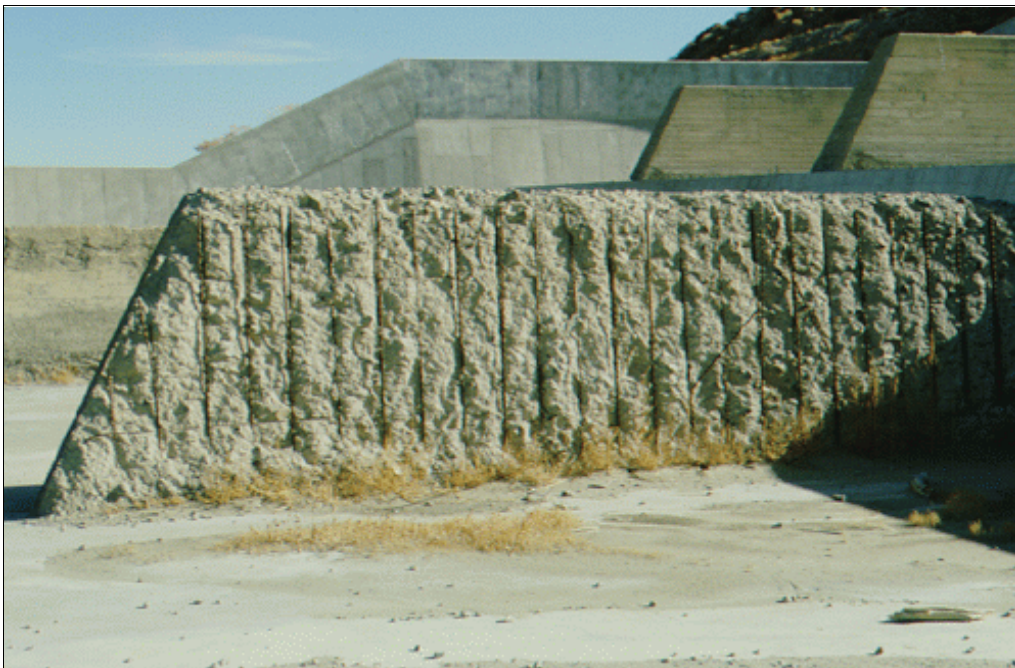
Figure 4.—This freezing and thawing deterioration should have been repaired before it advanced to the point that wall replacement or removal is the only option.
