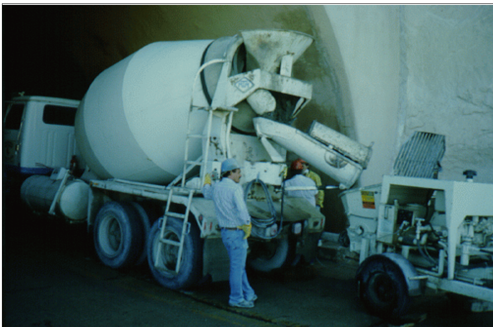
Figure 45.—Wet mix shotcrete equipment. The premixed shotcrete is delivered to the shotcrete pump by a transit truck.
