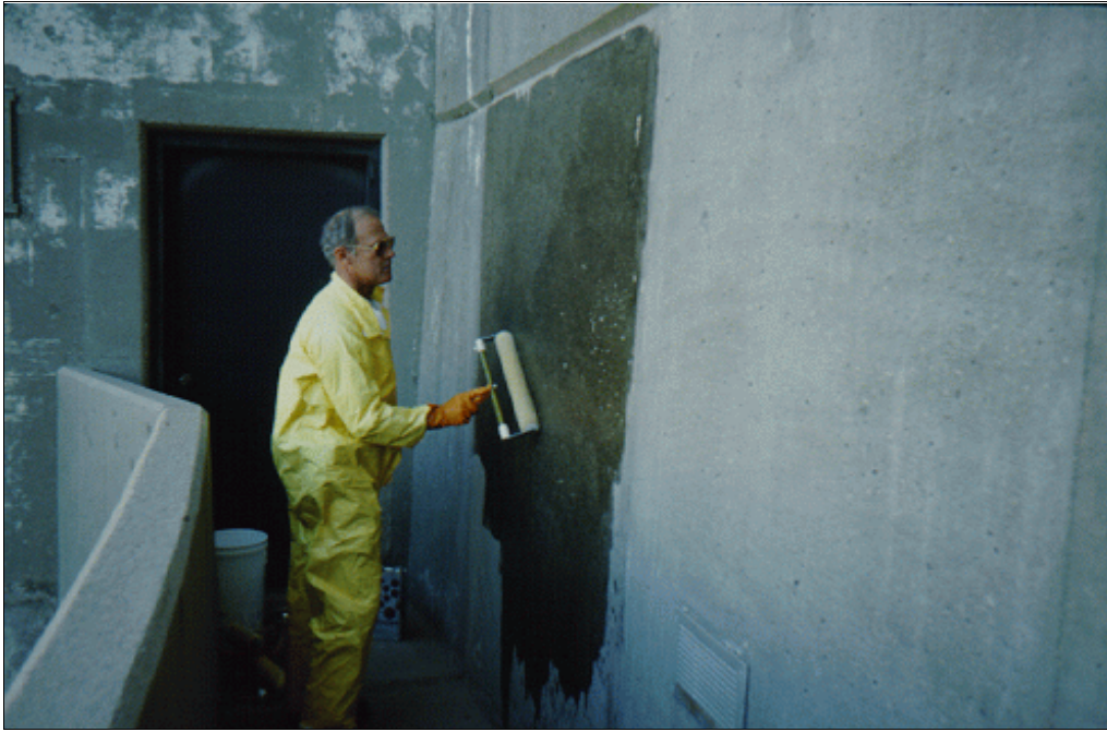
Figure 72.—A paint roller application of siloxane sealing compound to the downstream face of Nambe Falls Dam, near Santa Fe, New Mexico.
