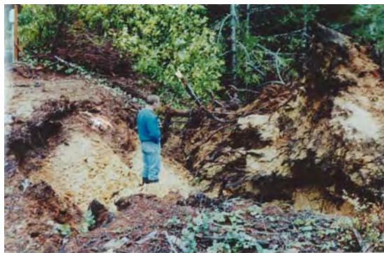
Figure 5. Serious damage by uprooted tree to embankment stability at a dam in Oregon.
