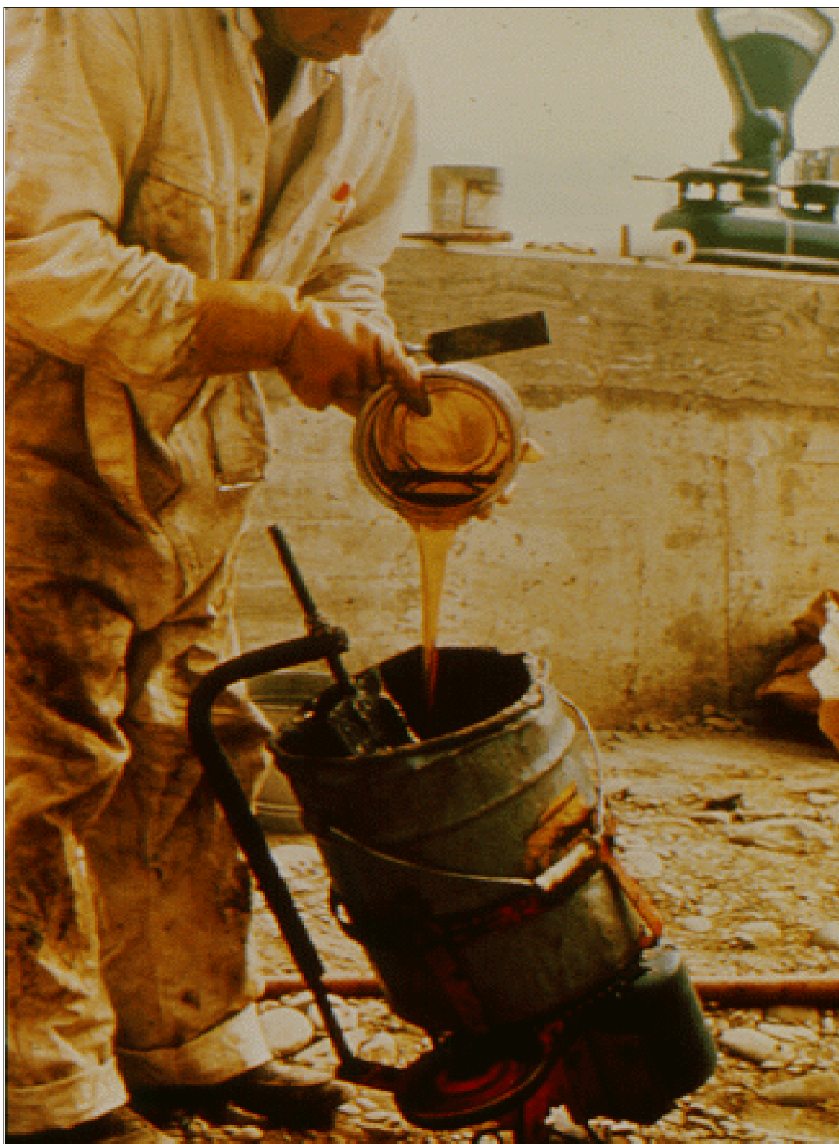
Figure 51.—A bucket mixer can be used to mix epoxy mortar for small repair areas.
