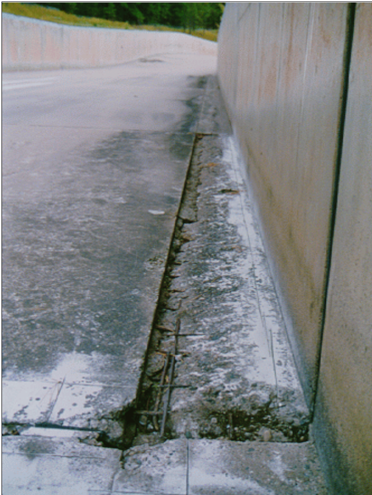
Figure 7.—This concrete damage was found to be a serious threat to the structural integrity of this spillway.
