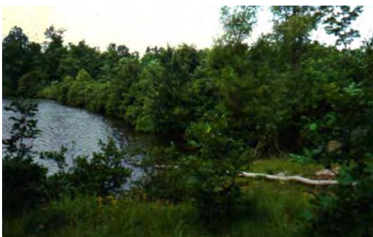
Figure 3. Example dam with inspection-hindering trees in Tennessee.
