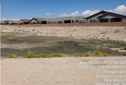
Ortav Albuquerque The pond side slopes are mostly bare dirt and will remain erosive until they are stabilized with rock armoring. The natural undisturbed condithion of the land is flat and not very erosive, but the steep slopes require a lot more cover to stabilize.
