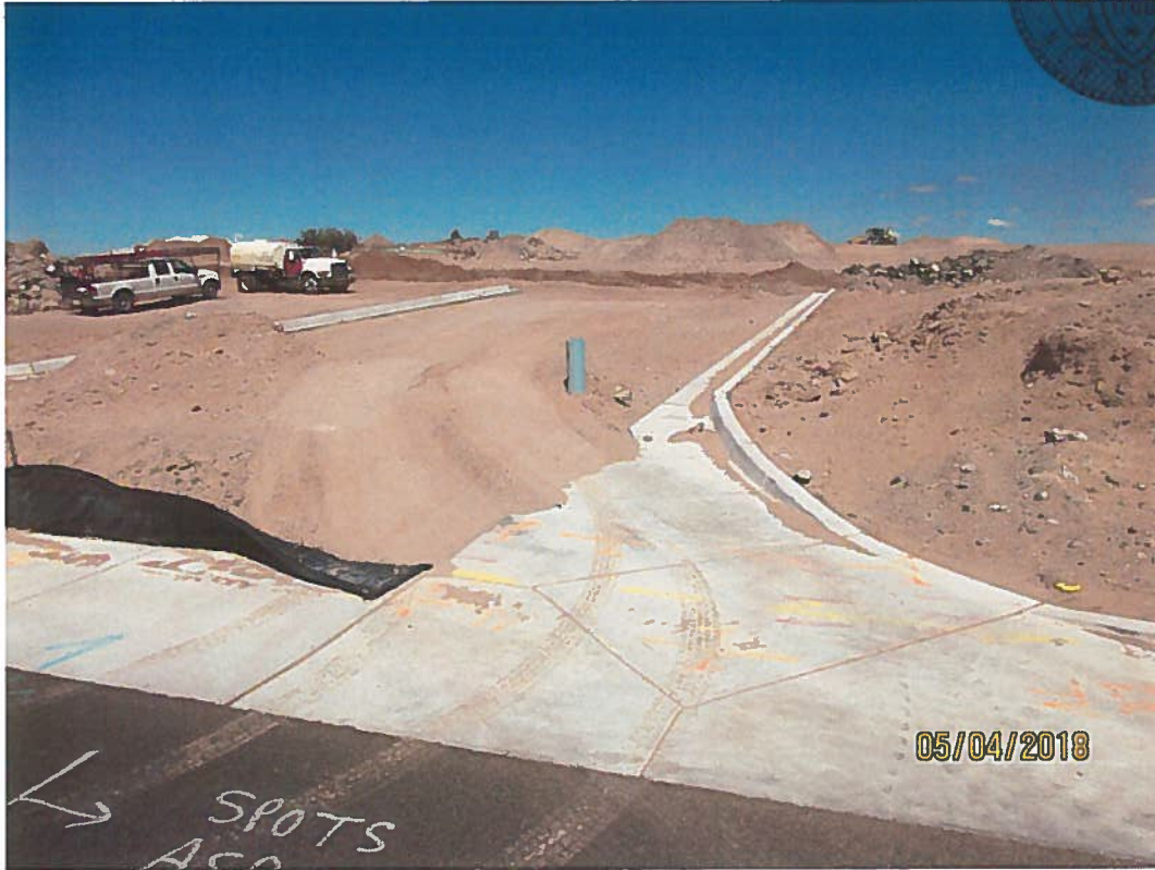
Workers exiting the site without vehicle tracking control. Sediment BMP required.
