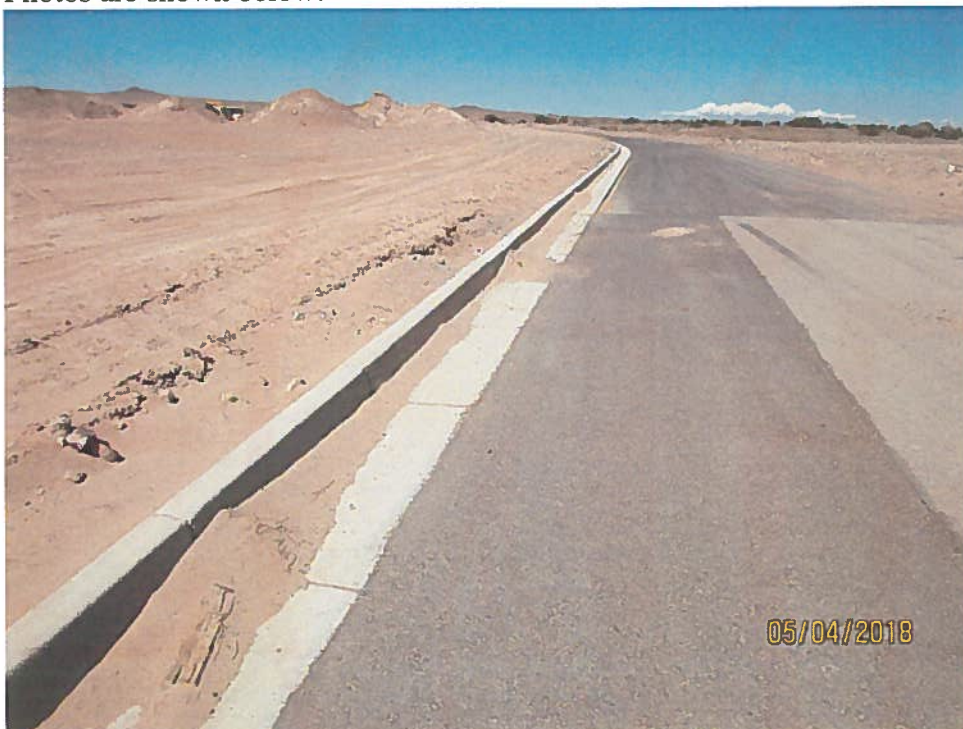
Sediment in gutter Rosa Parks Rd; south gutter.
