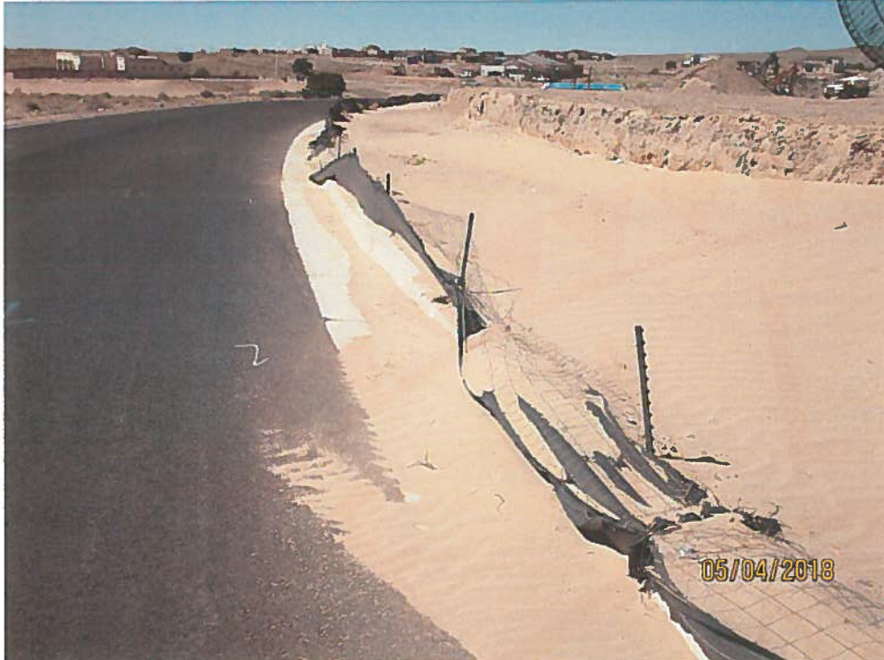
Silt fence in poor condition and sediment in Kimmick Dr.
