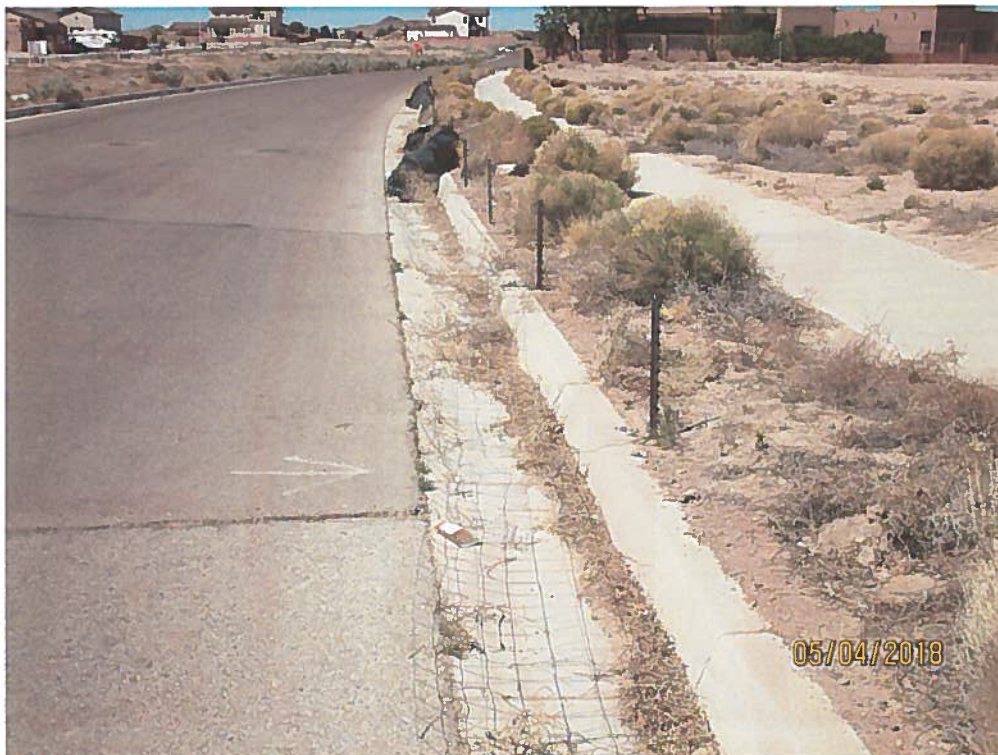
The remains of the silt fence have fallen/blown into the roadway.
