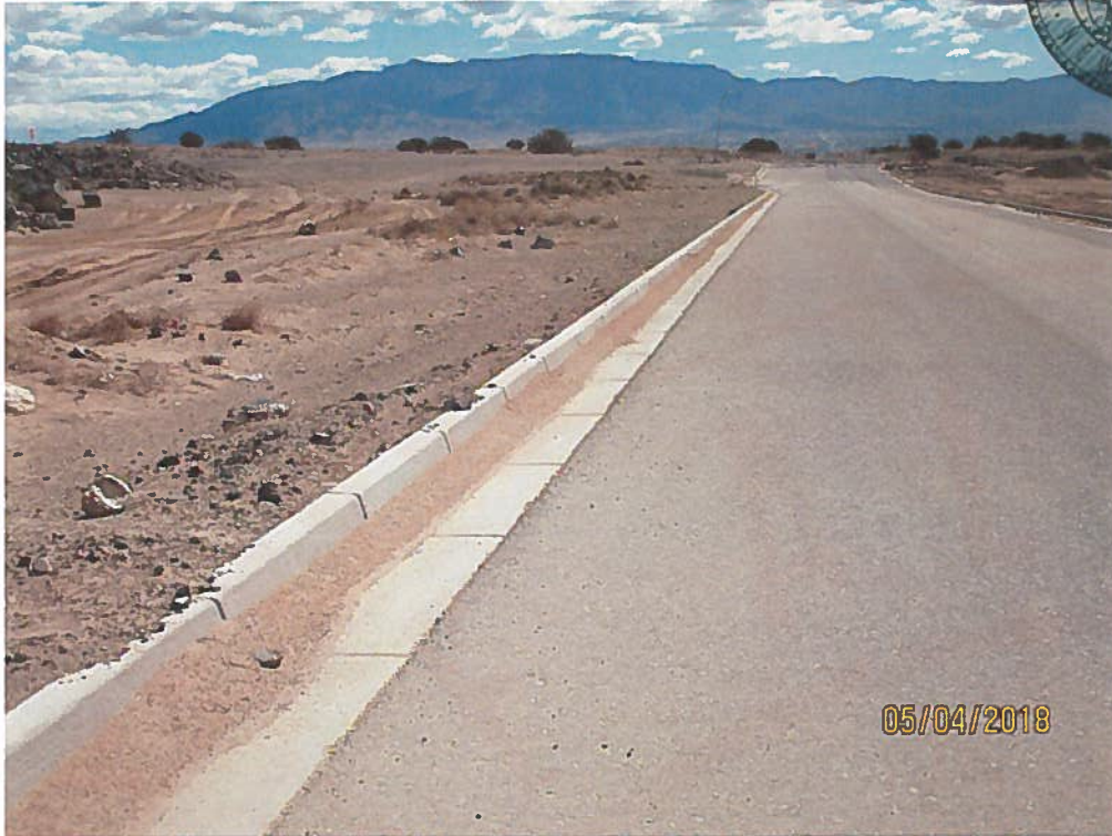
Sediment in gutter Rosa Parks Rd; north gutter.
