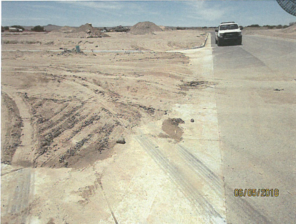
No Vehicle Tracking Control onto Rosa Parks Rd. Dirt on concrete apron of roadway.
