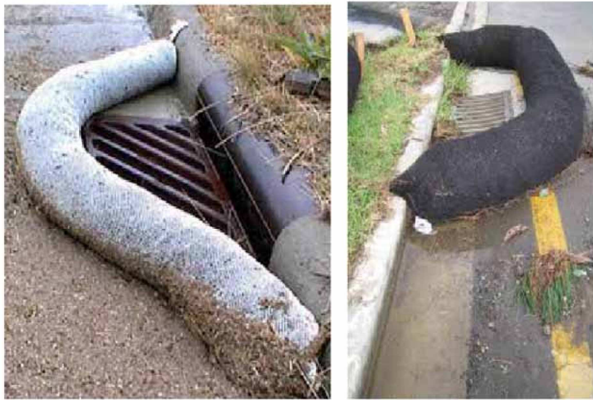
Curb Storm Inlet Protection with Wattles
