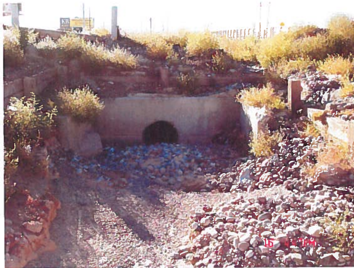
Existing 30" CMP that outfalls to the North Diversion Channel Between El Pueblo Road and the Railroad Tracks
