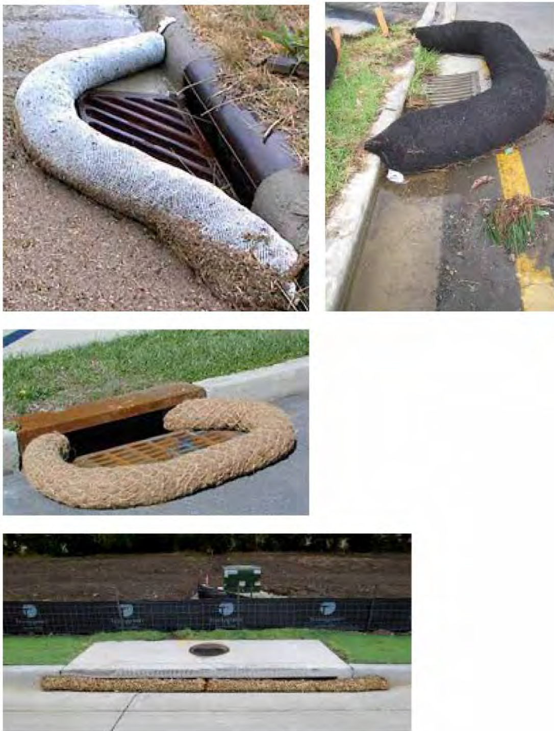
Curb Storm Inlet Protection with Wattles
