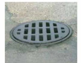
1. Remove sediment, debris, ice and snow from the inlet grate surface and surrounding area.
