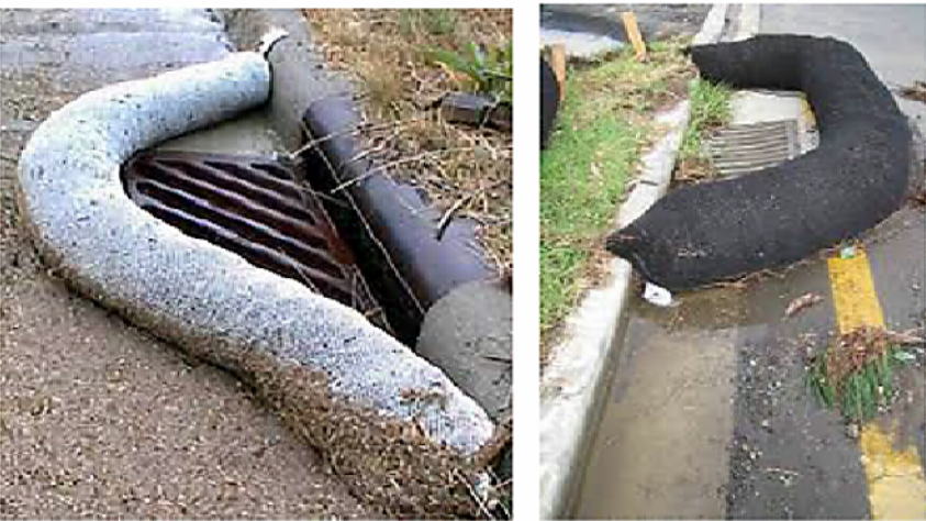
Curb Storm Inlet Protection with Wattles
