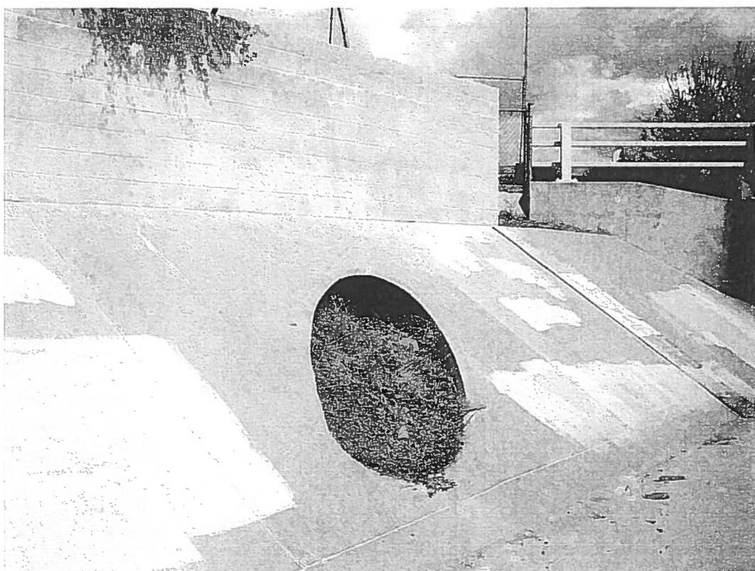
NORTH PINO ARROYO LOOKING EAST AT 54" STUB-OUT
