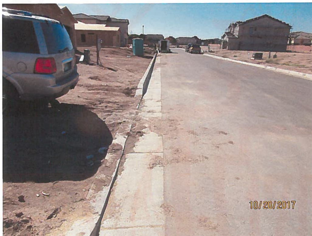
Sediment BMP required and sediment in street.
