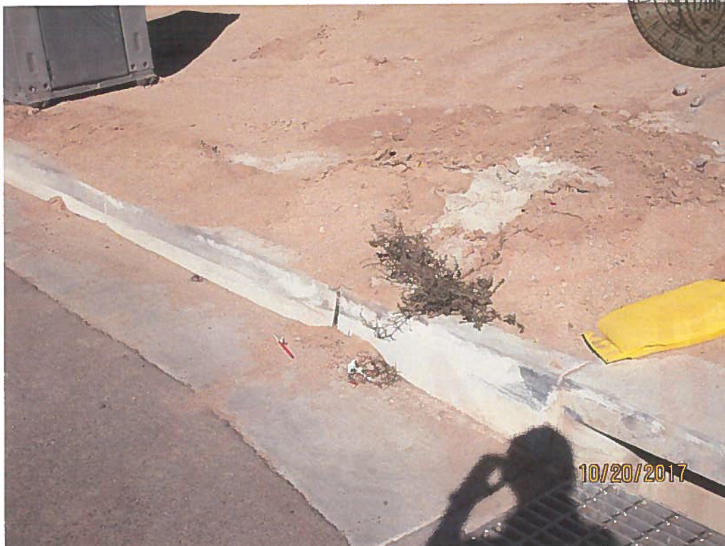
Sediment BMP required and sediment spilling over into gutter.
