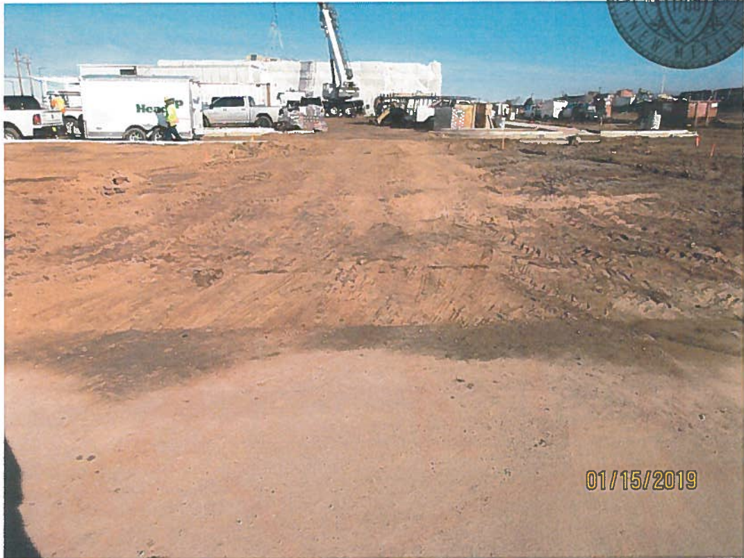
No Vehicle Tracking Control or sediment BMP.
