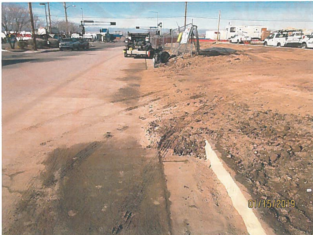
Sediment in street and dirt ramp in street/gutter.
