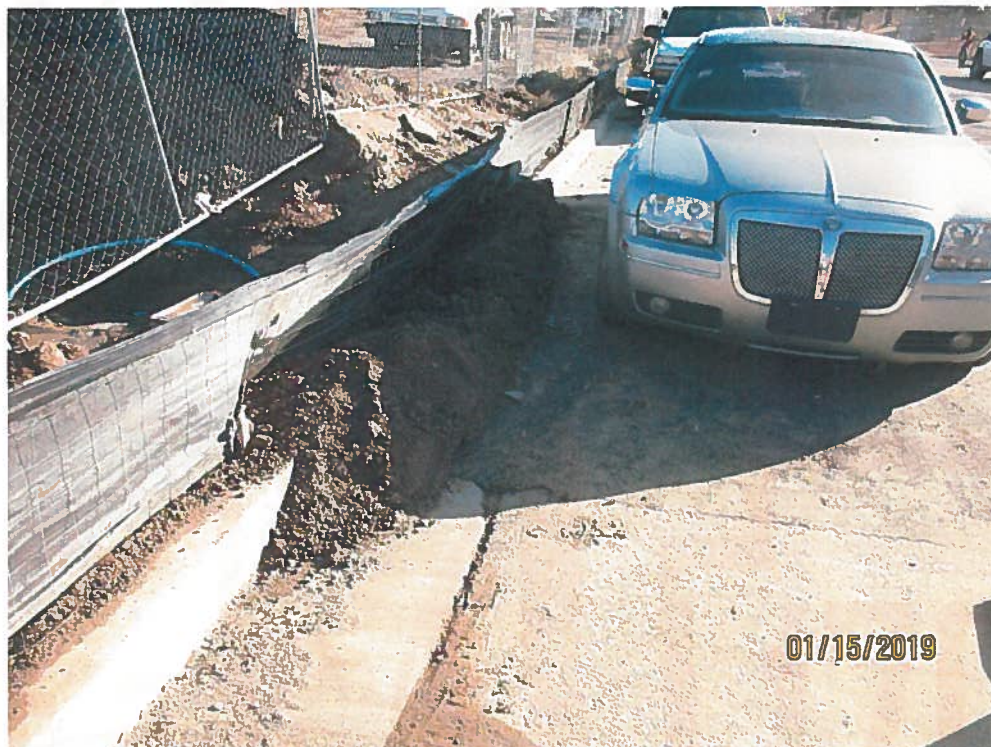
Dirt pile in the street with no sediment BMP.
