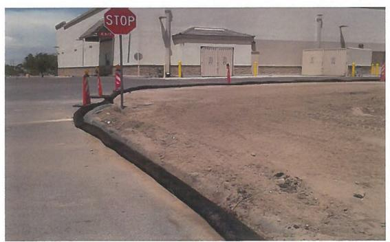
Item 3: On the south edge, a dirt ramp was built to get over the curb. This area drains to the channel that did not have a sediment BMP. A sediment BMP (rock bags or similar) the inlet to the channel would help catch it, but I advise to remove it as it will load-up the BMP faster than you want and maintenance will be required. A similar condition exists on the west edge. No ramp, but dirt in the drive aisle that drains to the channel. (Corrected, photo below)
