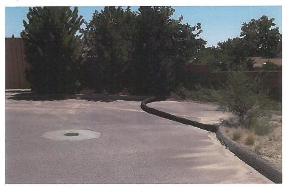
**Item 2**: In the NW corner, there was a gap in the filter socks and sediment washed through it. Please close the gap. This portion of the site is receiving offsite flows, which never helps. Also, there is a small dirt pile in the access drive outside the mulch sock. (Corrected, see photo below)
