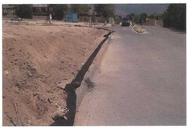
Item 4: There was a gap in the filter socks at the southwest corner and the dirt pile behind it is too high. (Corrected, photo below)
