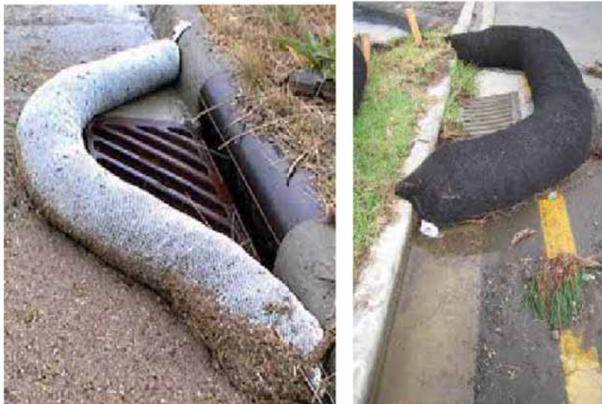
Curb Storm Inlet Protection with Wattles
