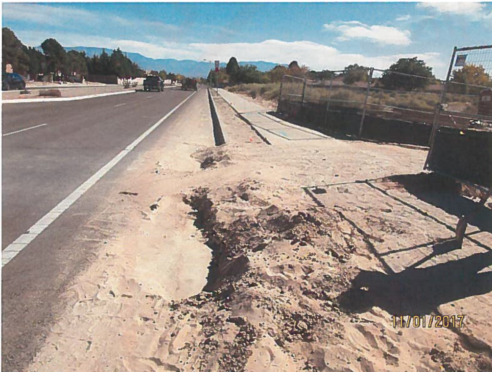
Dirt ramp in street, grade too high between sidewalk and back of curb and no track-out pad.
