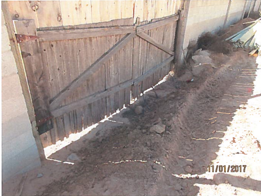
No sediment BMP at gate.
