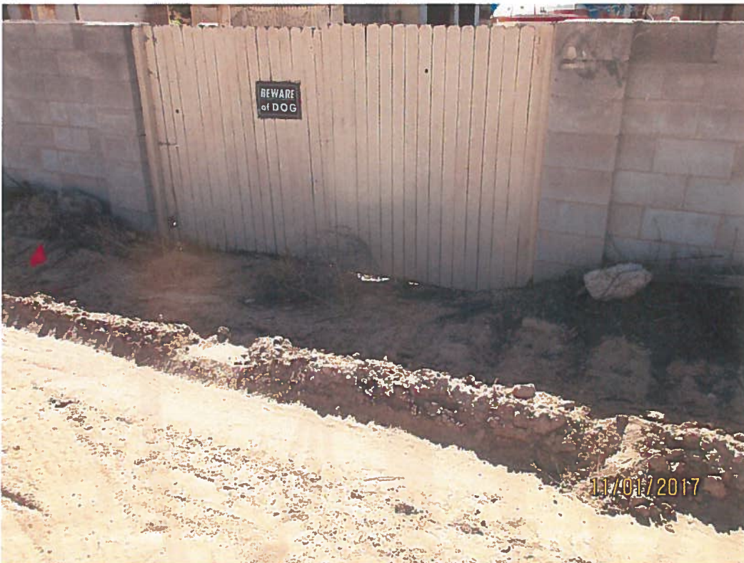
No sediment BMP at gate.
