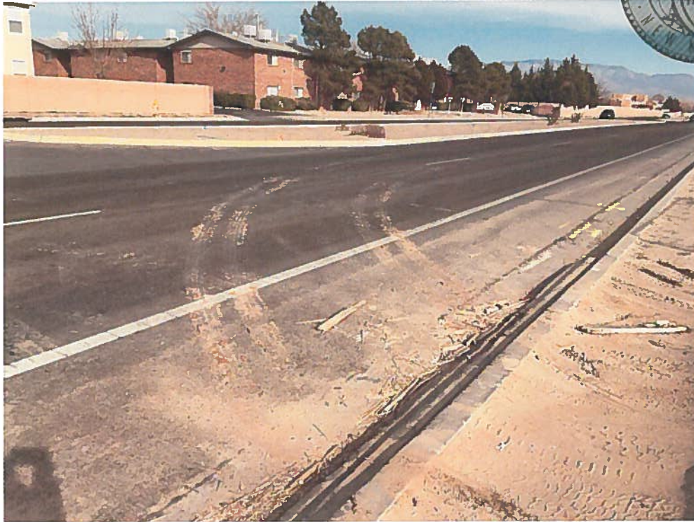
Track-out and wood debris on Montano Road.
