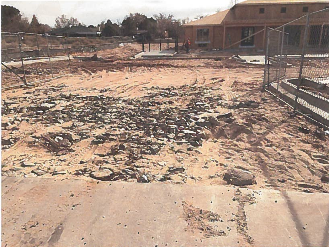
Track-out pad in poor condition.
